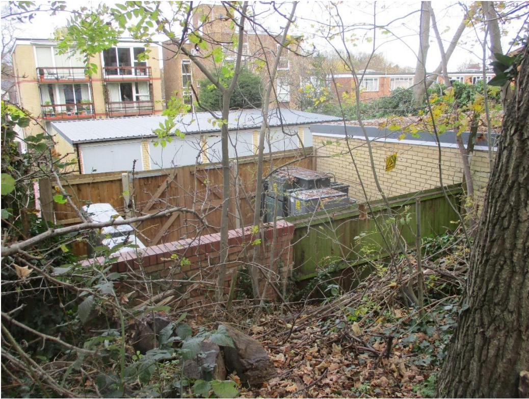
Photo 11: Photo of the electric substation located adjacent to the north east of the Site. Photo taken from the Site looking towards the north.
