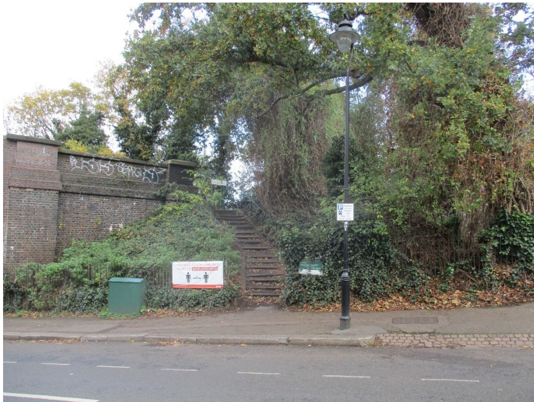
Photo 5: Pedestrian access steps from Stanhope Road to Parkland Walk. View from Stanhope Road looking towards the north east.
