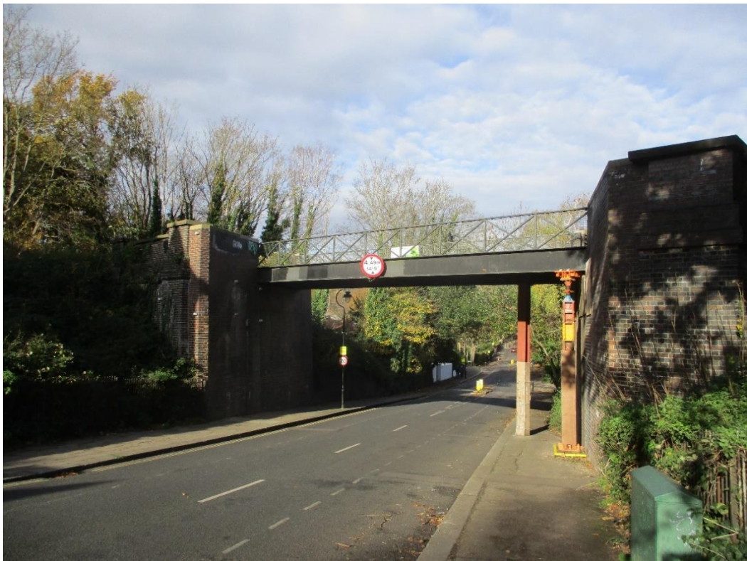
Photo 12: Bridge that crosses Stanhope Road. Photo is taken from Stanhope Road looking towards the north.
