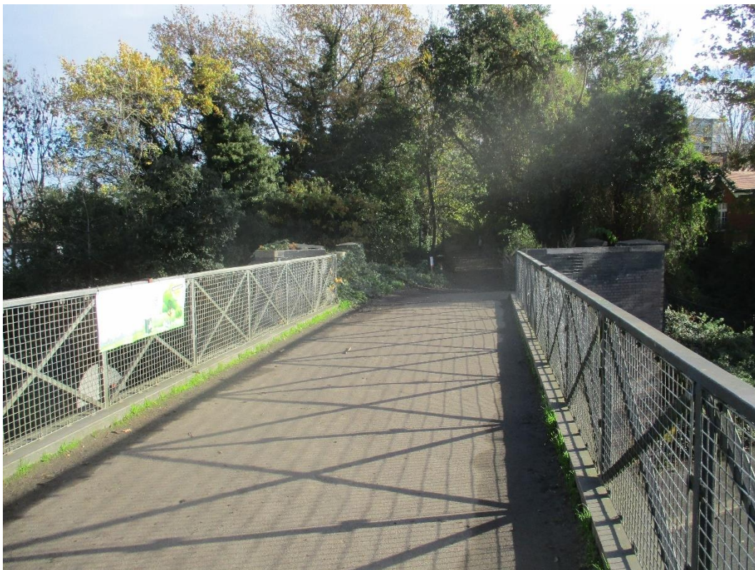
Photo 2: View of the bridge over Stanhope Road, looking towards the east.
