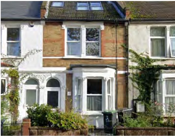
Yellow brick with red brick banding
