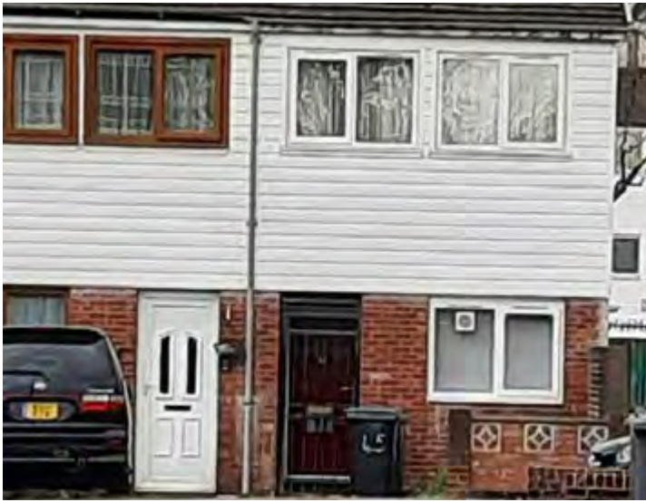
Wood cladding and red brick
