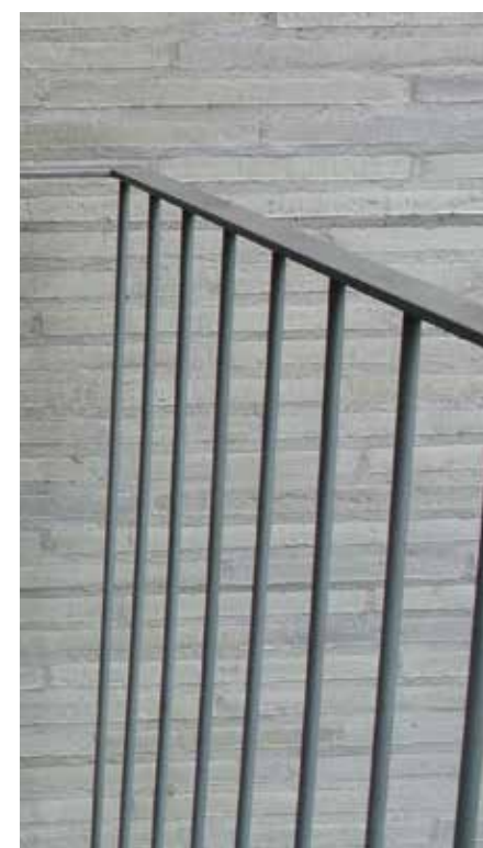
Painted metal balustrades
