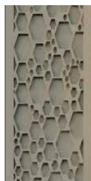
Perforated metal screen to acoustic ventilation panel
