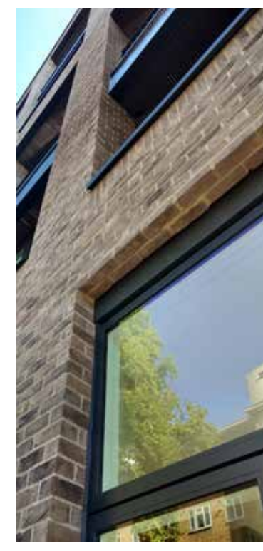
Proprietary black PPC aluminium glazing system
