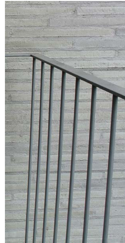
Painted metal balustrades
