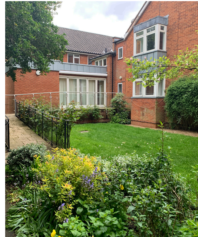
Unsympathetic extension to Kekewich House.
