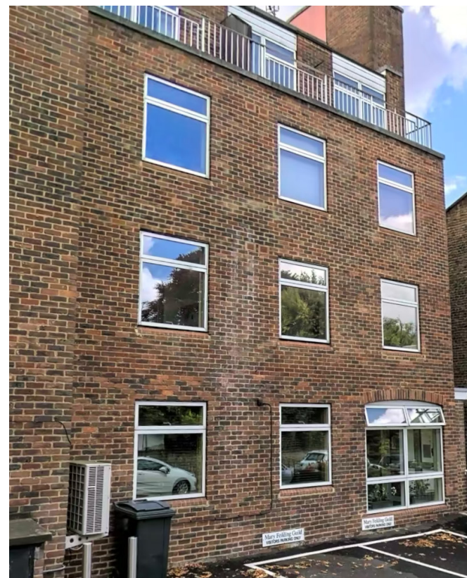
Truscott House Facing North Hill.
