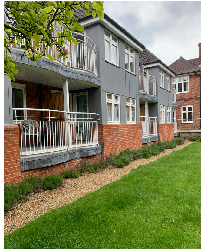
Contemporary extension building at rear garden.
