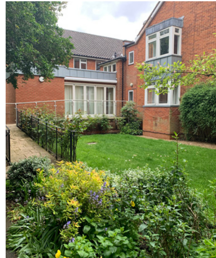
Unsympathetic extension to Kekewich House.
