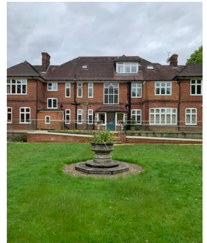
Rear of Kekewich House.
