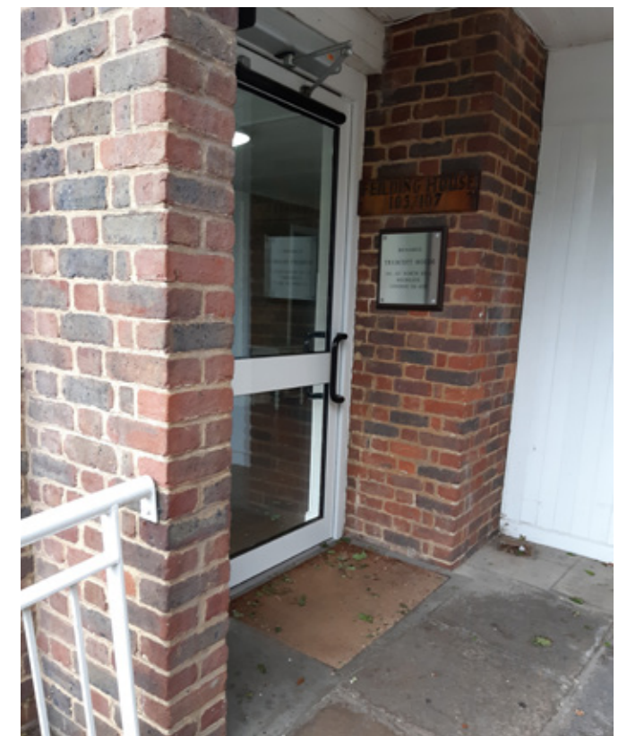
Existing main entrance at Truscott House.
