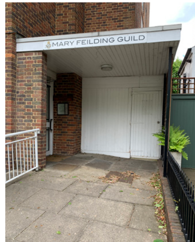
Existing main entrance at Truscott House.
