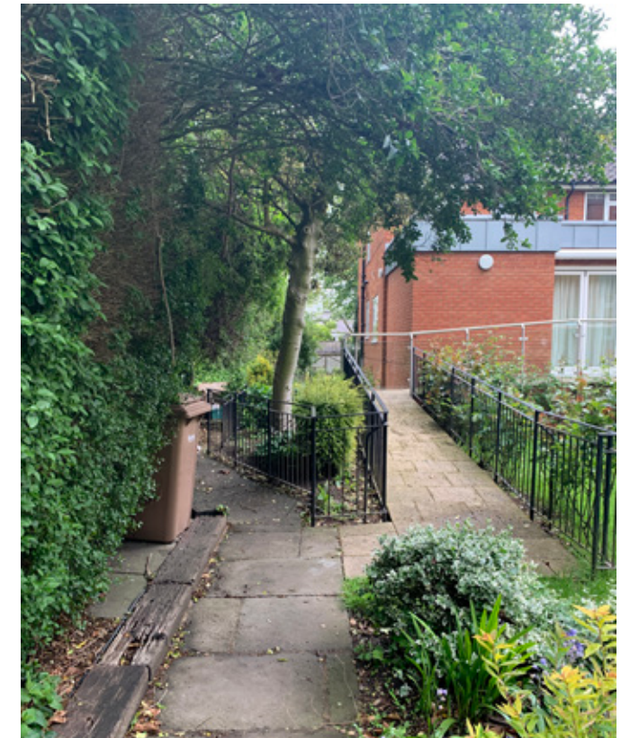
Existing ramped access to extension building.
