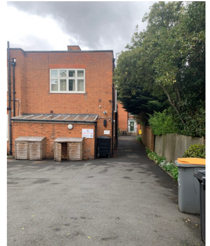
Unsympathetic extension to Kekewich House.
