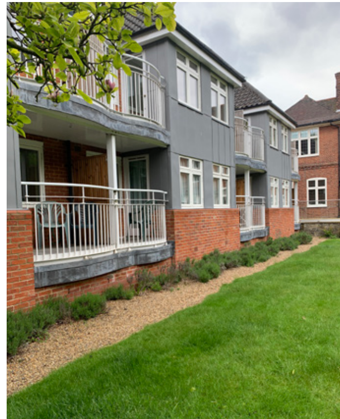
Contemporary extension building at rear garden.
