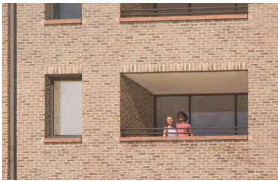
Recessed balcony framed by terracotta coping and soldier course lintel
