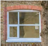
Terracotta expressed openings
