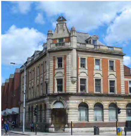
Fig. 127: Chamfered London Corners High Road, Tottenham
