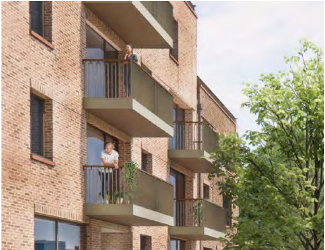
Fig. 111: Projecting balconies overlooking the courtyard
