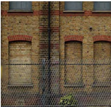
Recessed blind window with expressed lintel Electrical substation, Church Lane
