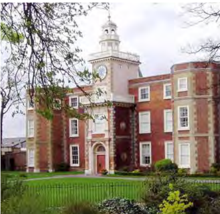
Railings, Bruce Castle Park
