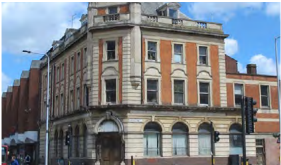
Chamfered London Corners High Road
