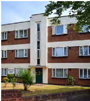
Landscape format windows Bruce Castle Court (Locally listed)
