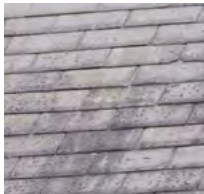
Peabody Cottages slate roof
