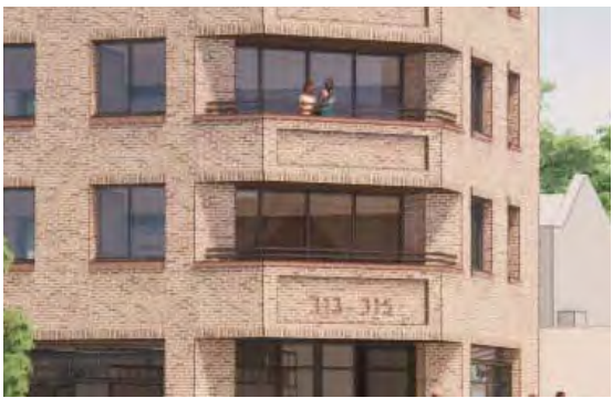
Chamfered corner with terracotta precast sill Indent to brick
