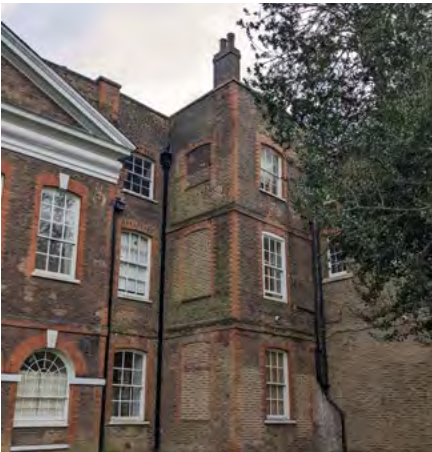
Fig. 124: Blind windows on the Northern Elevation of Bruce Castle
