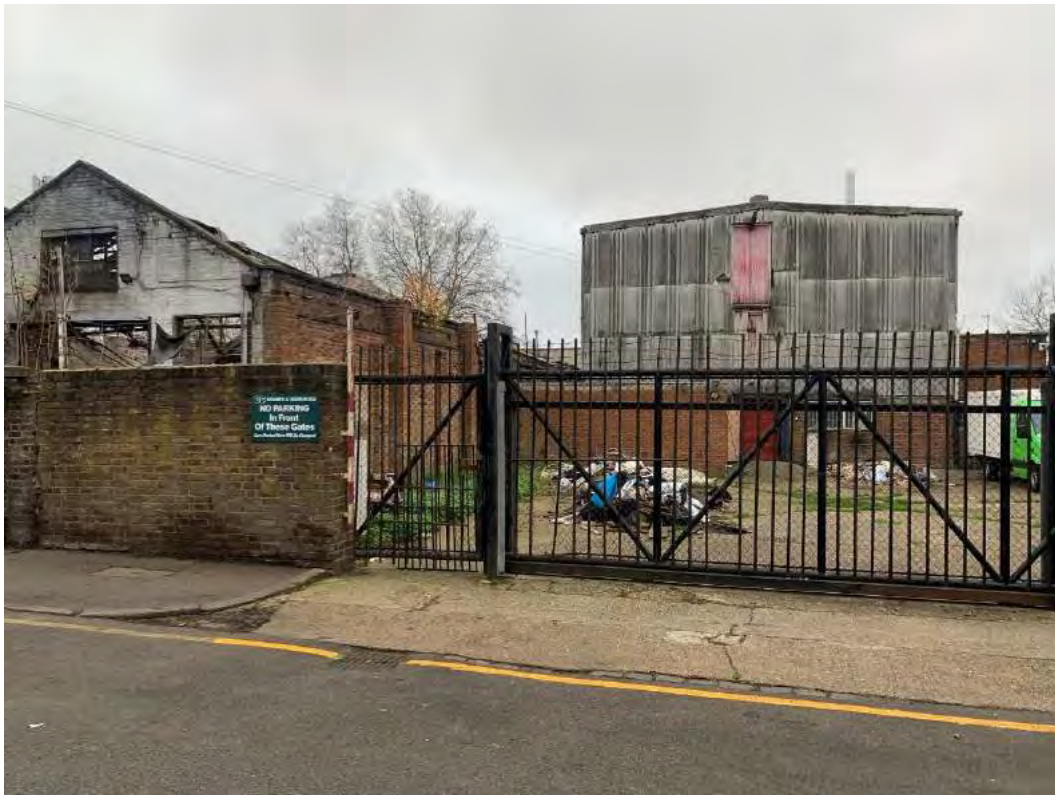
Figure 2-6: Existing Footway Conditions along Church Lane
