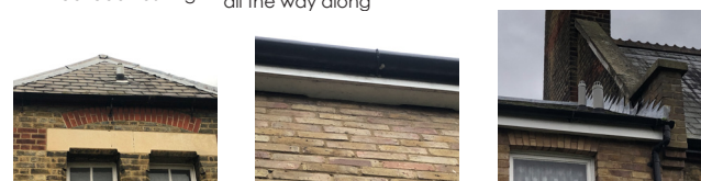
Lifted lead flashing
