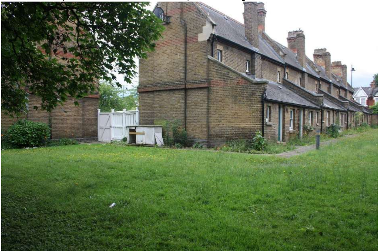
Plate 16: Development area for new north-west corner pavilion looking south.
