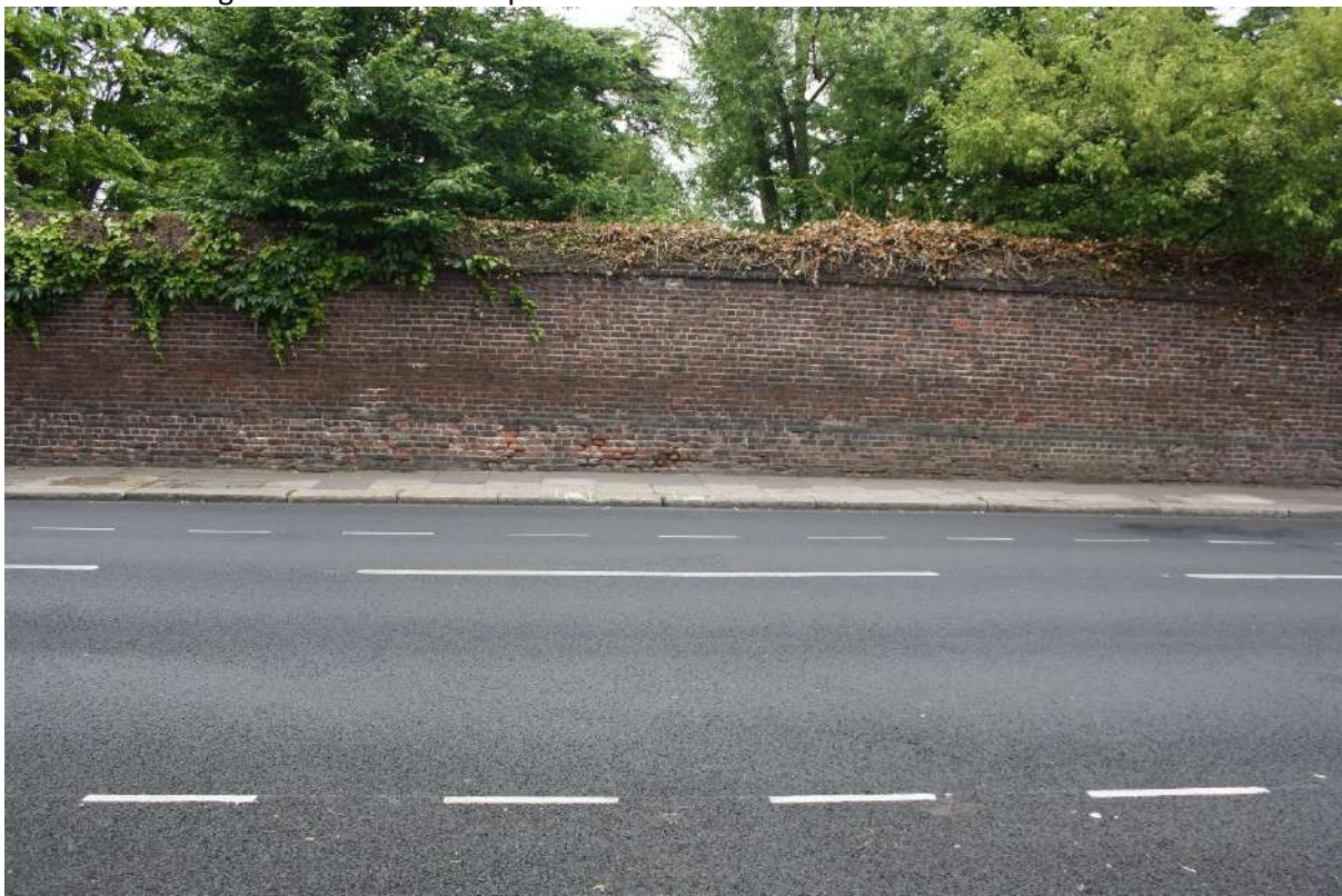
Plate 34: Looking north-west from Site boundary with Lordship Lane, to South boundary wall To Bruce Castle Park.
