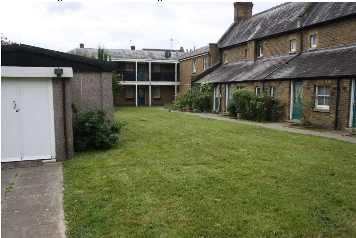
Plate 26: Looking south-east towards building to be demolished.
