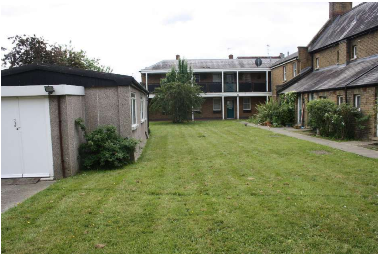
Plate 25: Looking south-east towards building to be demolished.
