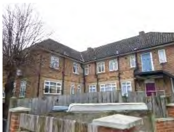
Photo 6. Rear elevation of B10.
