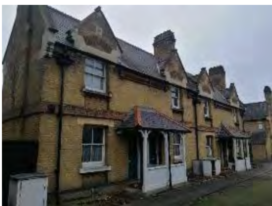
Photo 3. Typical front elevation of almshouses.
