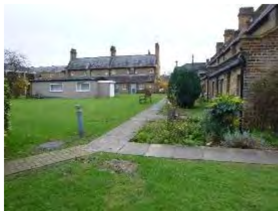
Photo 2. Rear gardens and B9.
