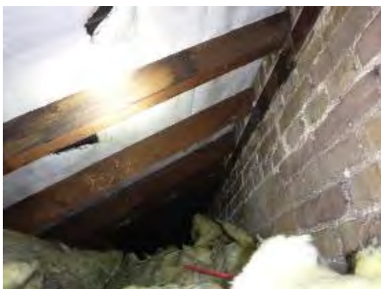
Photo 5. Loft space above lean-to extension.
