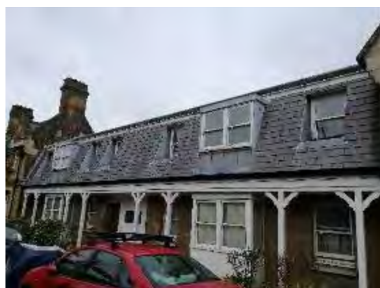
Photo 4. 70s infill building (B7).
