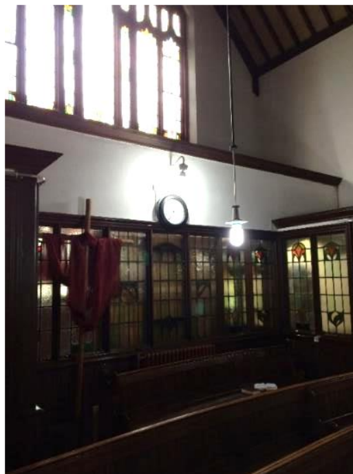
Figure 4.9: Showing the vestibule to the northern side of the church.
