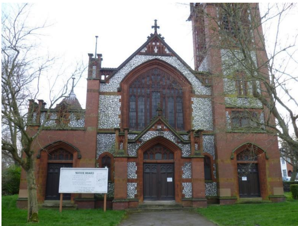
Figure 4.6: Northern elevation (autumn/winter) with no leaf coverage to trees adjoining front elevation 1
