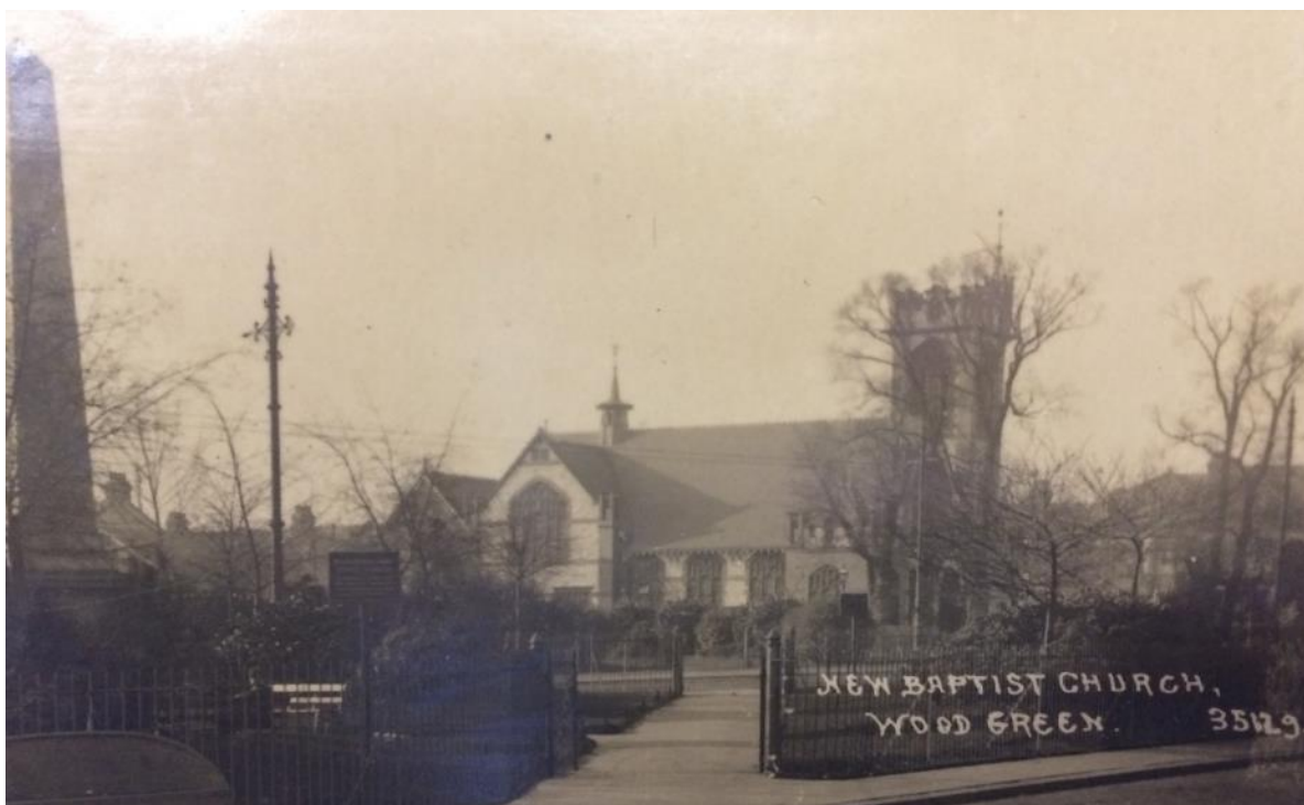
Figure 5.1: Braemar Avenue Baptist Church, Braemar Avenue. Source - Haringey Local Archive, Bruce Castle Museum. The photograph is undated but appears to be from the interwar period.
