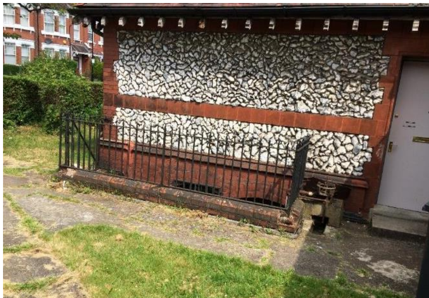
Figure 4.4: Railings and dwarf plinth wall to the stairs to the basement plant room.
