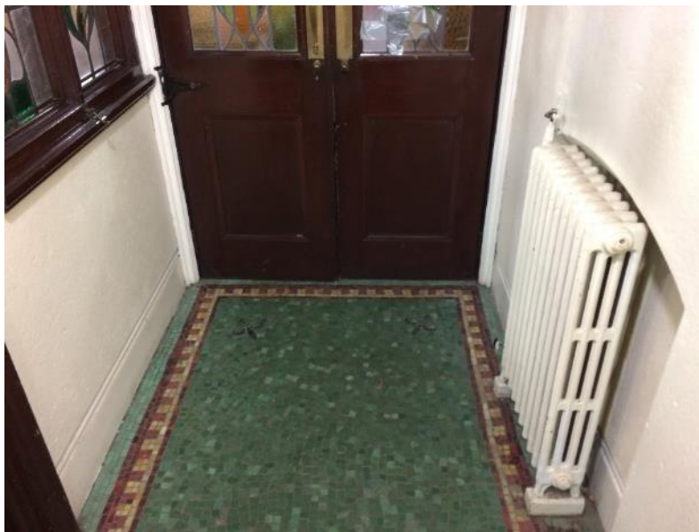
Figure 4.10: Original mosaic tiling, cast iron radiators and part panelled doors to front entrances.
