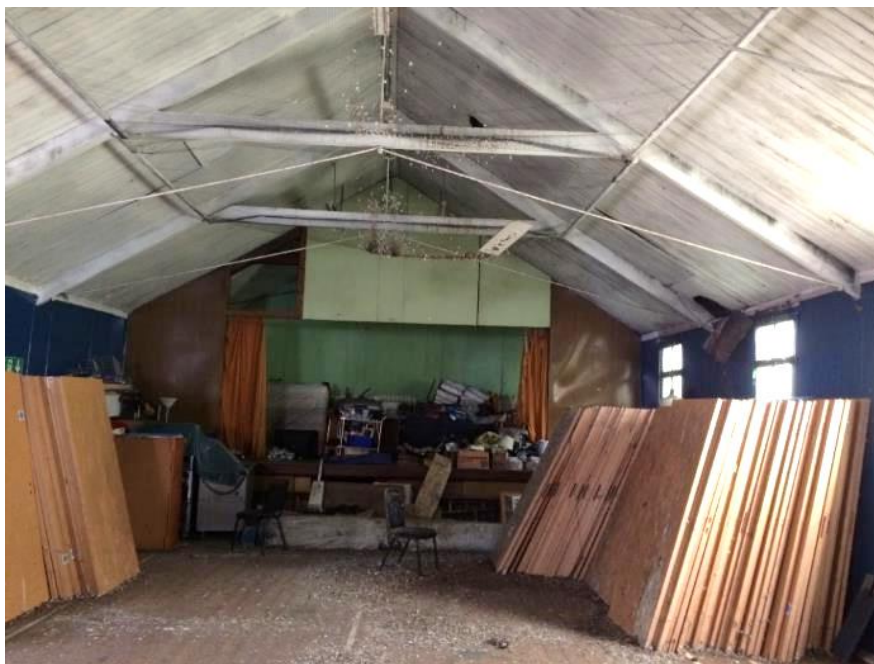
Figure 4.30: Hall interior looking east.
