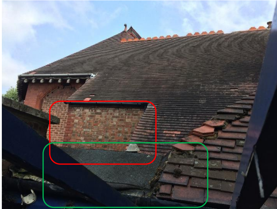
Figure 4.3: Showing two sections of roof amended when the 1950s extension was added. Beyond to the left is the blocked window.
