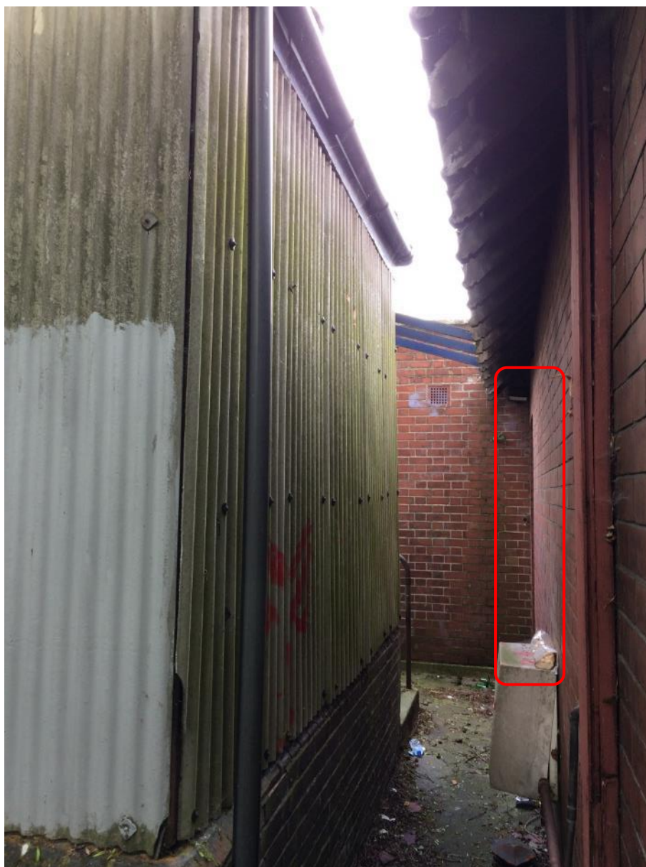
Figure 4.5: Southern elevation of church to the right-hand side, modern extension in the centre and the church hall to the left-hand side. Junction of the original church and 1950s extension marked in red.
