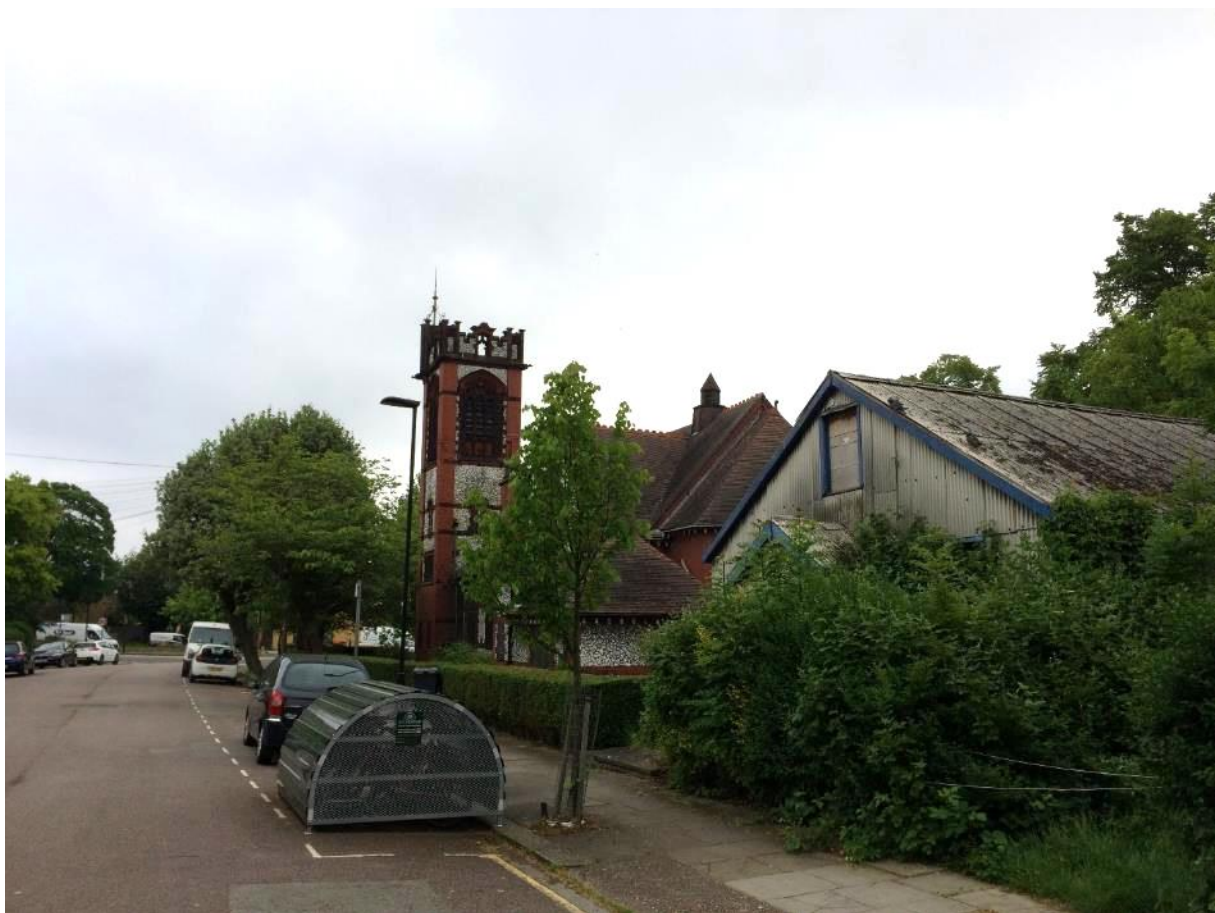
Figure 4.1: Western elevation of the church, with the church hall to the south, right hand side.
