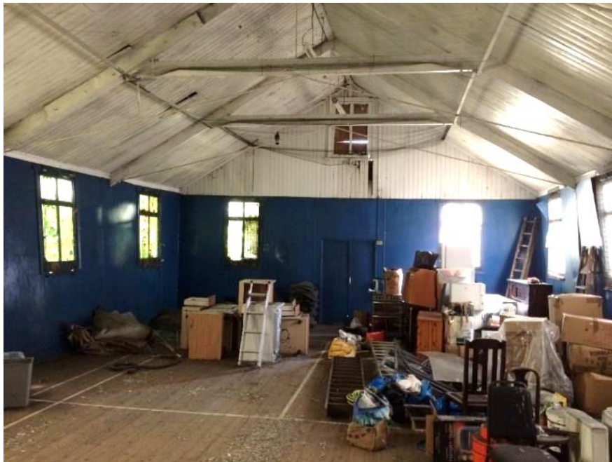
Figure 4.29: Hall interior looking west.
