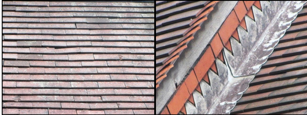
Photographs 7 - 8: Close-fitting roof tiles & valley flashing
