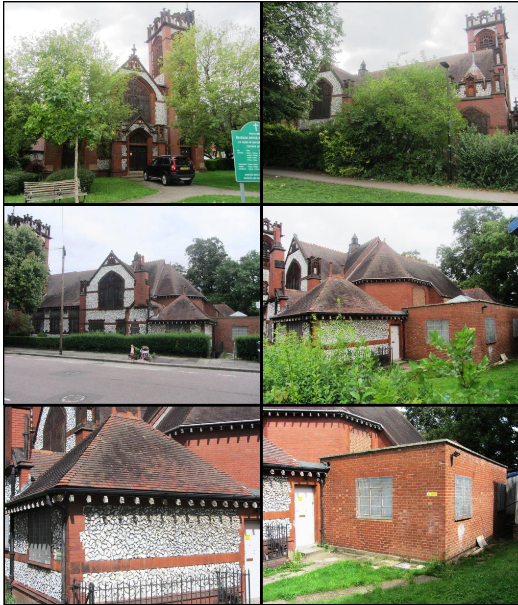
Photographs 1 - 6: Braemar Avenue Baptist Church - front, rear & side elevations
