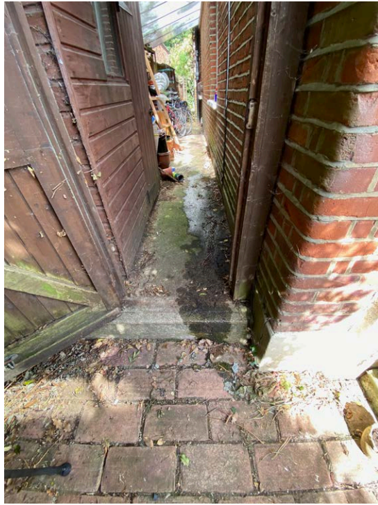
View of the side alley from front elevation.
