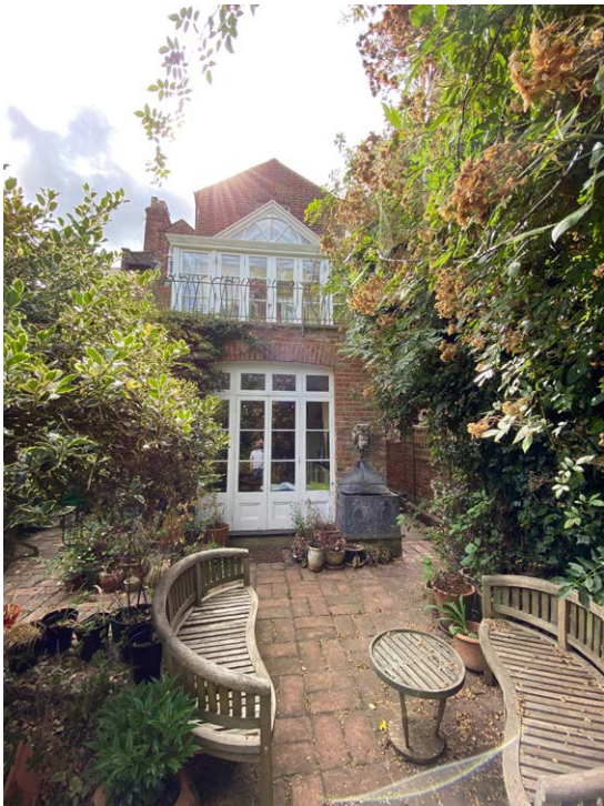
View of existing rear elevation.
