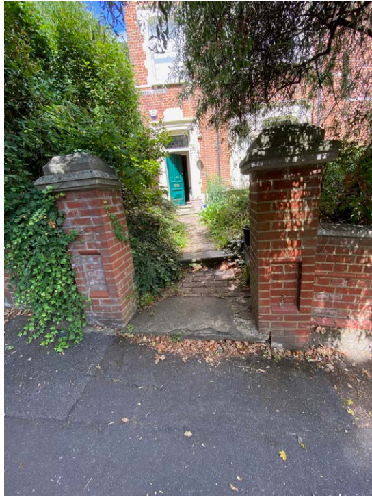
View of the Front elevation from street
