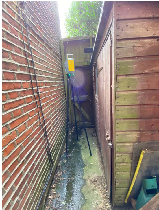
View of existing fence and side access, and existing shed.
