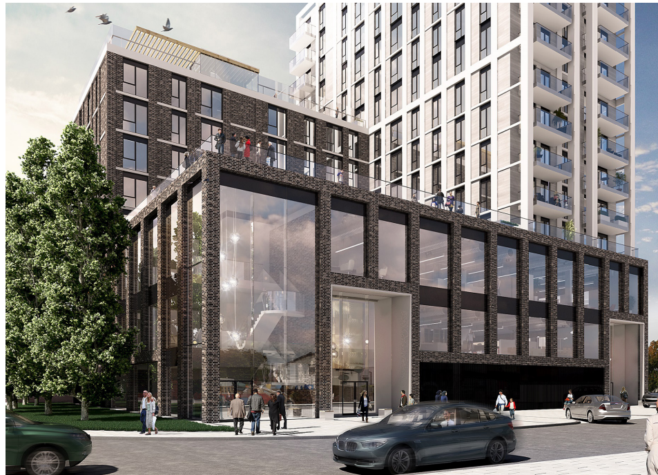
SIMPLE BRICK FRAMING TO BASE
