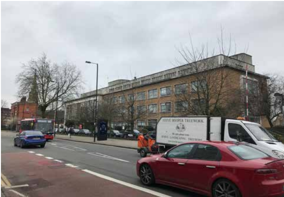
Figure 5.2 View of the principal façade of Haringey Civic Centre from the High Road (note this photograph dates from 2020 and does not show the full extent of exterior façade deterioration)
