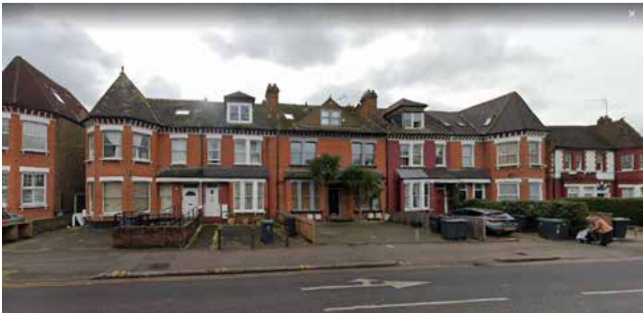
Figure 5.4 Residential development along Bounds Green Road
