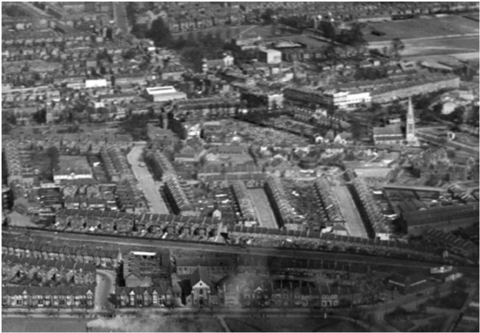
Figure 4.2 Extract from aerial view of the area taken in 1930 with St. Michael's Church and the Fishmongers' and Poulterers' Institution Almshouses visible (Source: Britain from Above, ref: EPW031496)
