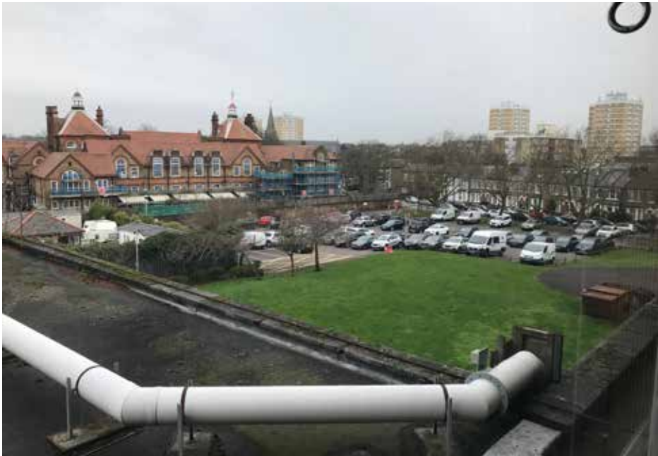
Figure 5.3 View of the car park to the rear of Haringey Civic Centre
