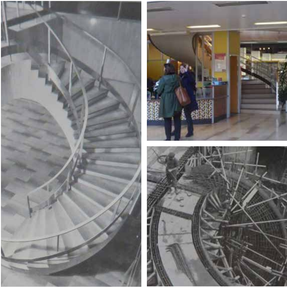
Figure 3.8 Images of the helical main staircase under construction (Architect and Surveyor, 1958), completed (Architect and Surveyor, 1958) and with existing reception desk installed (2018)
