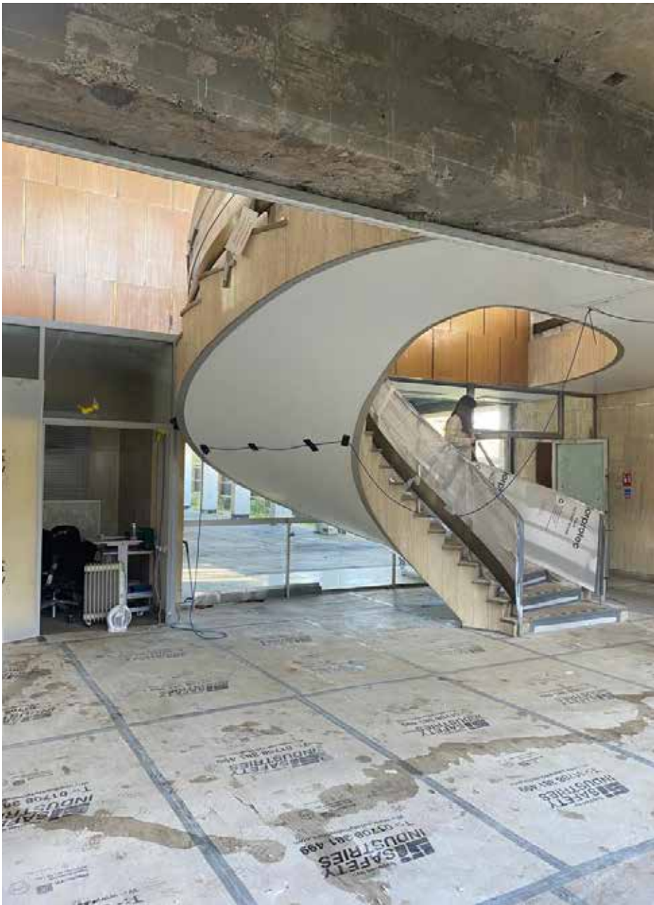
Figure 3.22 Image of the soft strip of the main reception and staircase.
