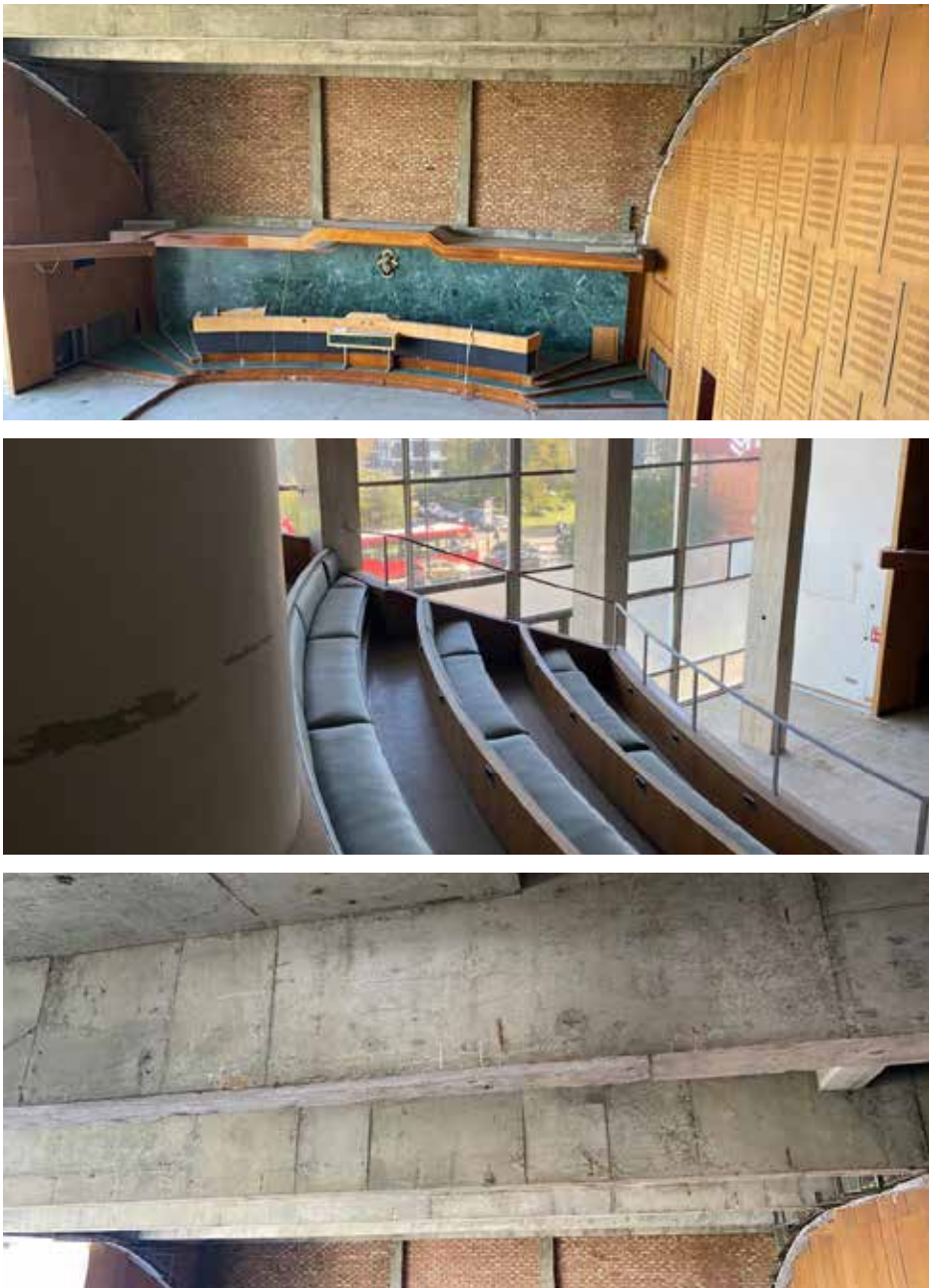
Figure 3.21 Image of the Council Chamber with the asbestos ceiling now removed.
