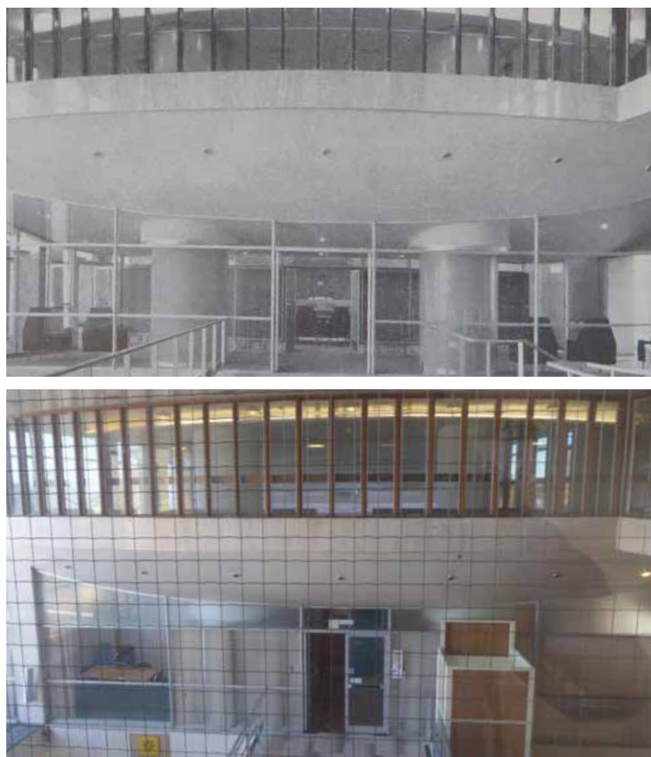
Figure 3.9 Image of bridge to entrance of the Council Chamber in 1958 (Architect and Surveyor, 1958) and existing with wheelchair lift visible (2018)
