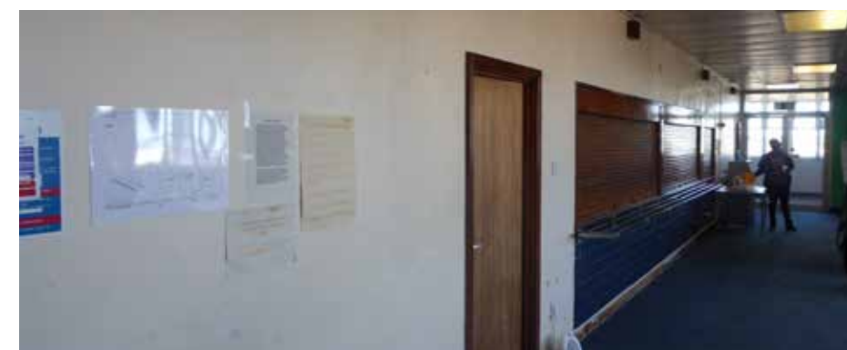
Figure 3.17 Image of third floor canteen in 1958 (Architect and Surveyor, 1958) and as existing (2018)
