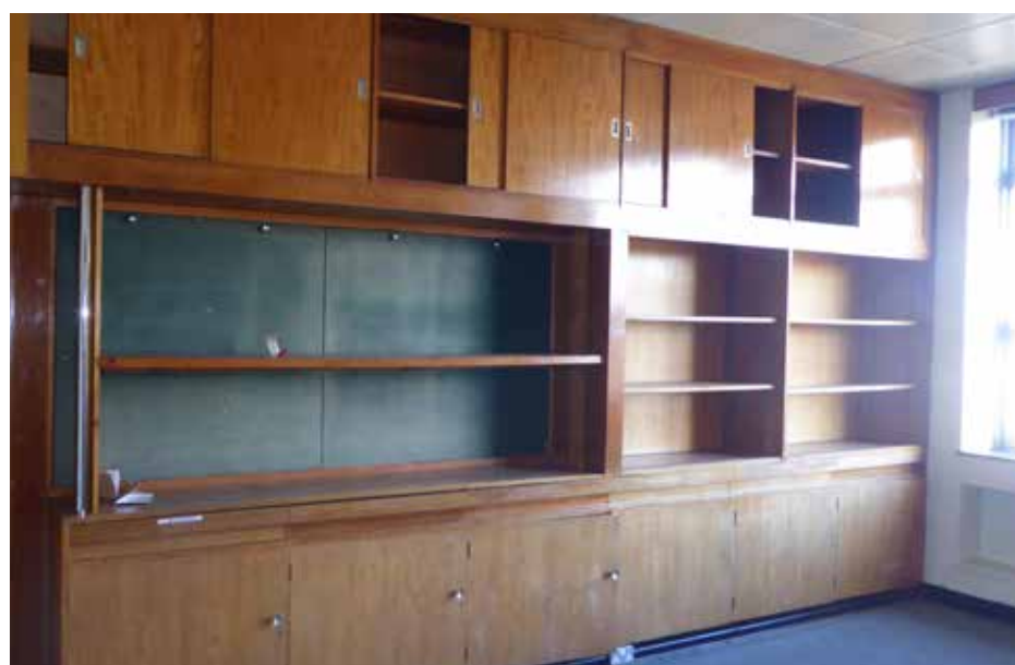
Figure 3.13 Image of second floor office interior taken in 1958 (Architect and Surveyor, 1958) and as existing (2018)
