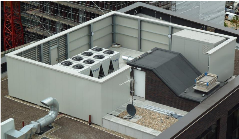
Figure 6—4 Mechanical plant noise barriers
