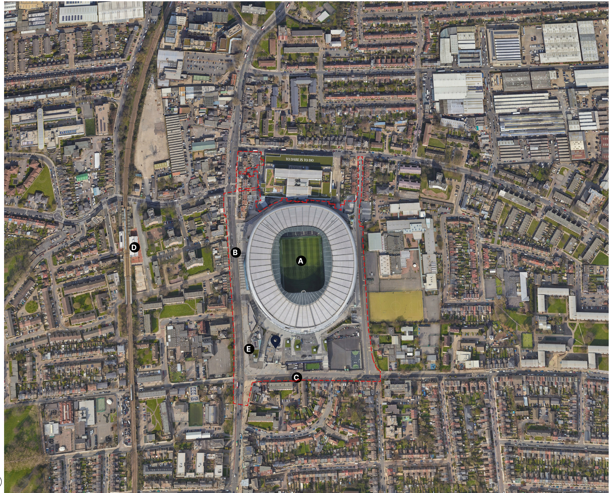
FIGURE 2. Site Aerial Overview
