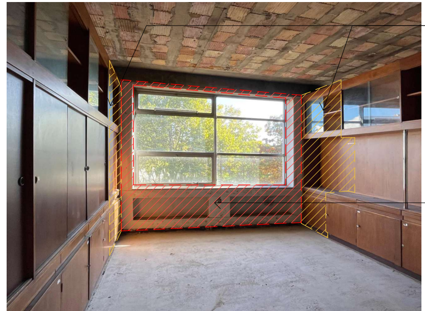
Existing External Wall Condition - Heritage Joinery/fitted furniture
