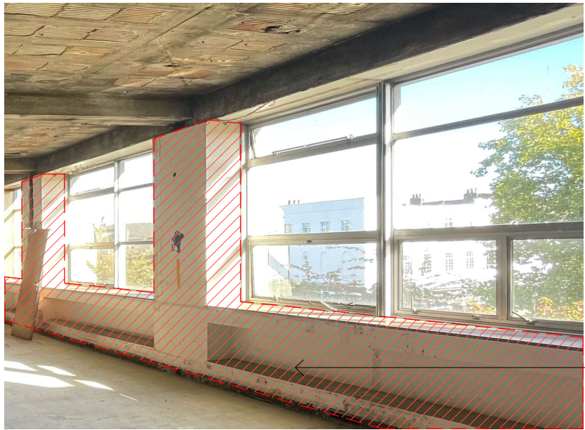
Existing External Wall - General condition
