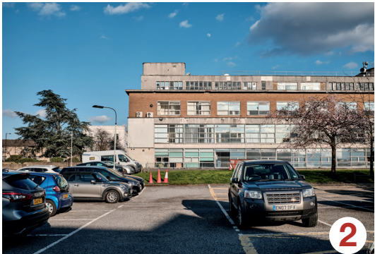
Car Park Site
