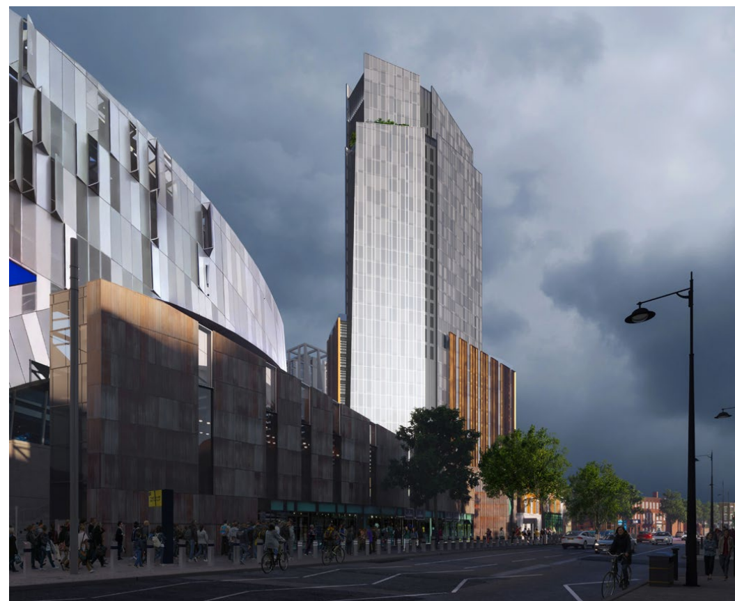
FIGURE 75. View from the High Road Looking South
