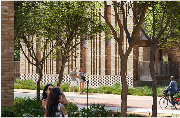
perforated masonry to allow carpark ventilation
