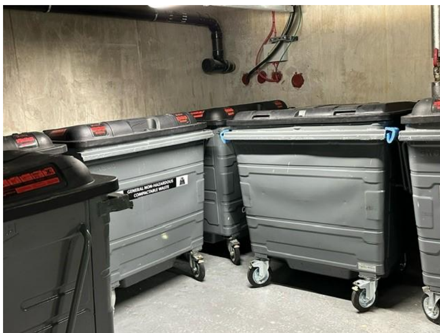
General waste bins have signage on them stating 'General Non-Hazardous Compactable Waste'.
