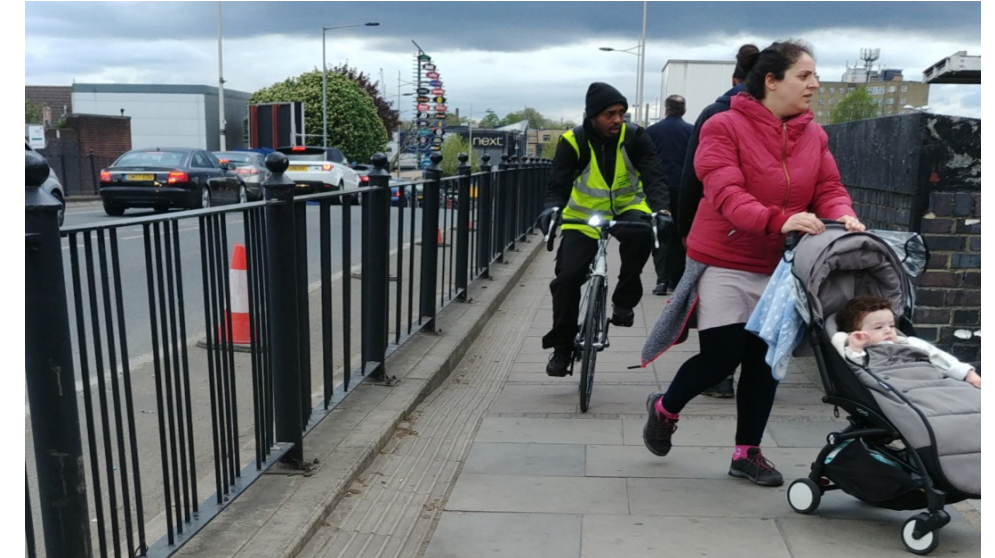
Eastern end of Ferry lane bridge, looking west over the bridge, showing the highly constrained space for pedestrians
