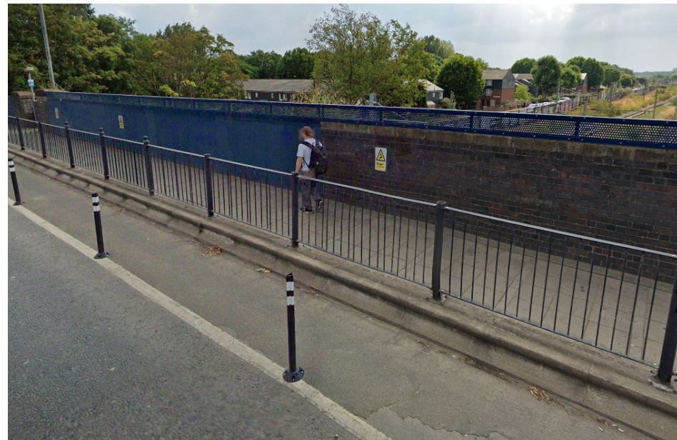
On Ferry Lane bridge showing the Trief kerbs that are required to protect the bridge structure and the guard rail to stop pedestrians crossing in unsafe places. Image Google Street View
