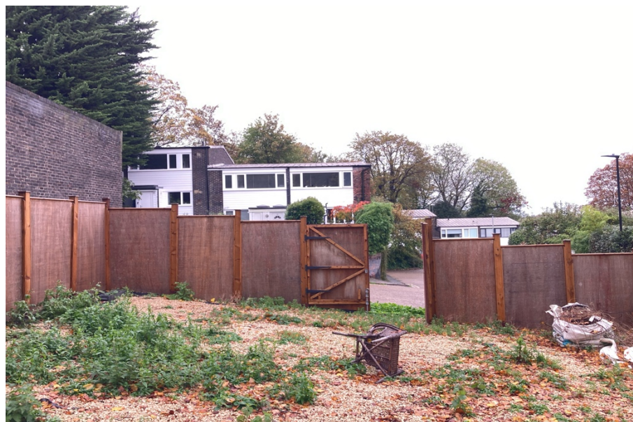
Figure 6 Internal view of site, showing hardstanding and the land now devoid of trees, with high boarded fencing enclosing the land for security purposes. Note that dumping continues to take place despite the fencing.
