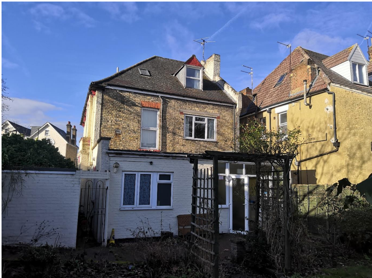
Figure 3 Existing property, looking from the garden at the rear
