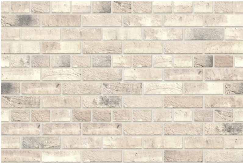
Brickwork: Medium grey stock brick, stretcher bond with light grey mortar.
