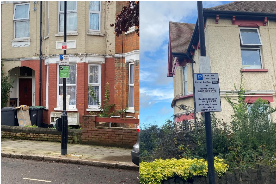
Figure 3a & 3b: Electric Vehicle Charging Point along Maryland Road & Woodside West Controlled Parking Zone
