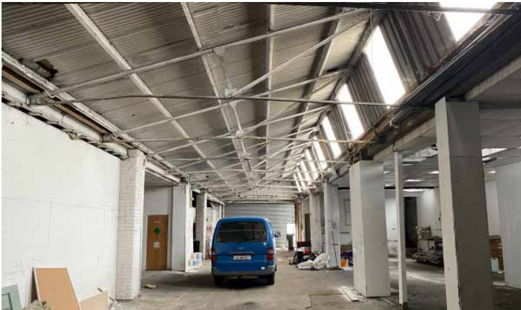
View 7- Inside of the existing building
