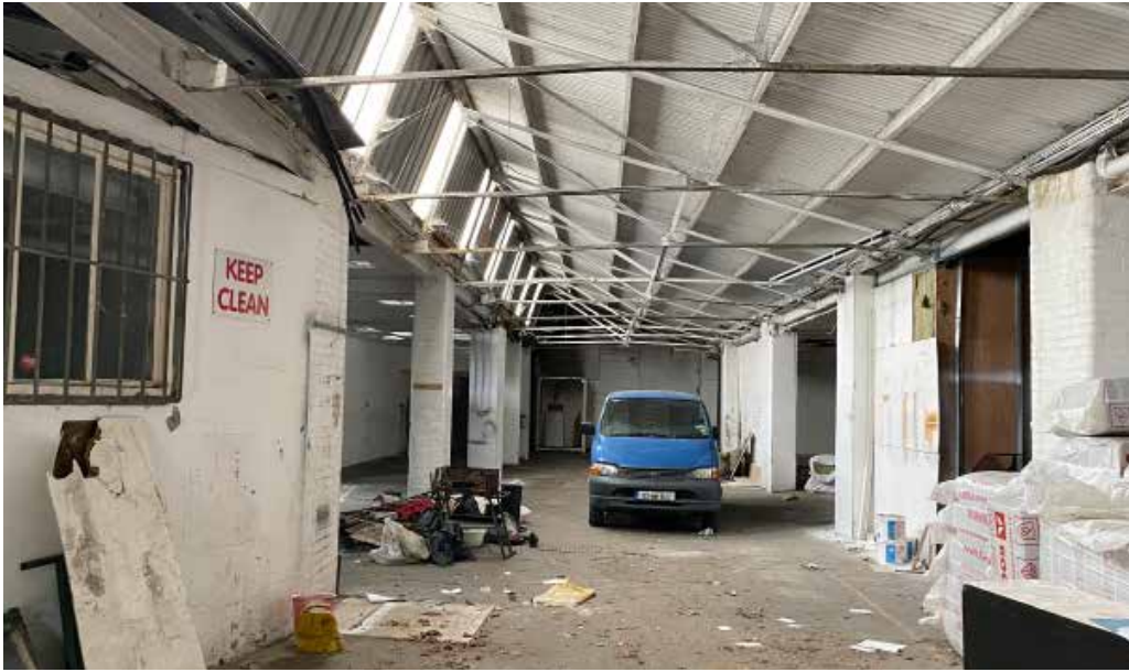
View 8- Inside of the existing building
