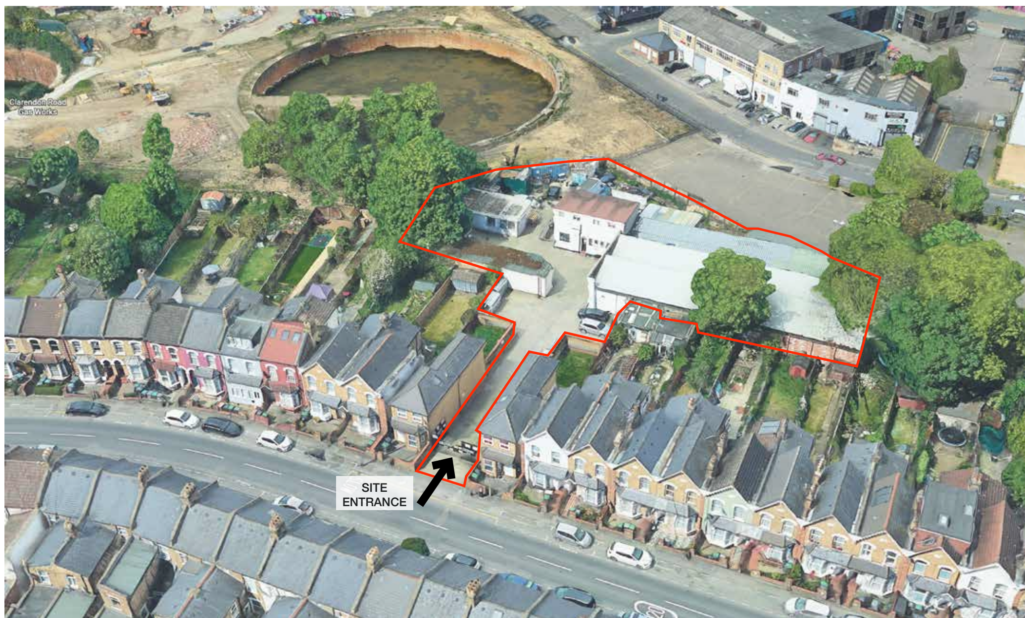
Overview of the Site as seen from the east
