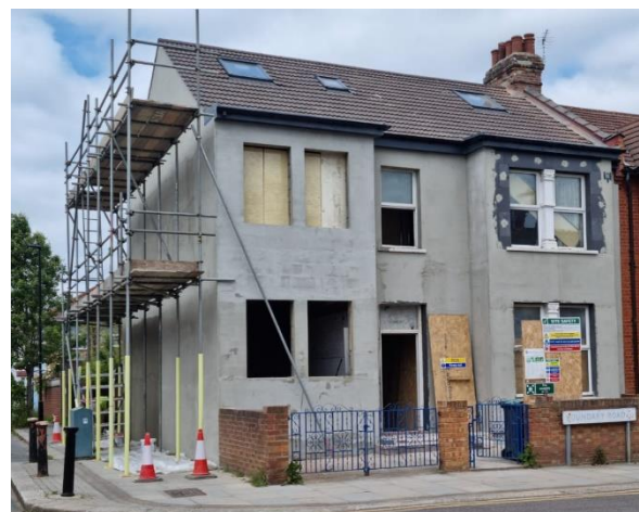
2-storey side extension under construction
