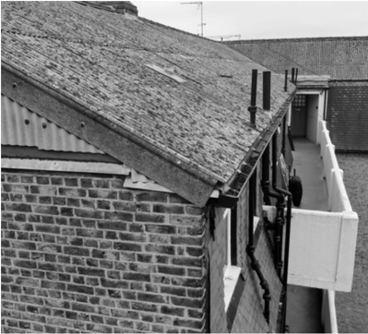
A - View looking at the rear garden north west corner
