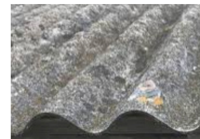
Corrugated Chrysotile sheet roofing
