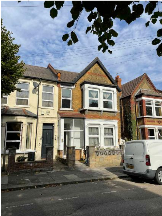
A VIEW OF THE FRONT OF 11 NORTHBROOK RD
