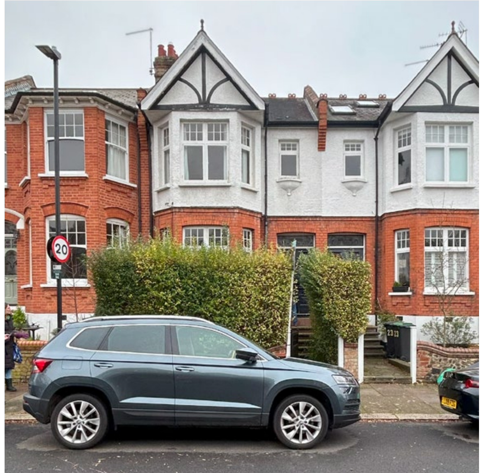
Photo of existing building on 21 Thirlmere Road
