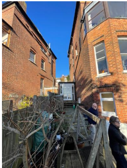
3. Photograph of the Existing 60/62 Side Extensions
