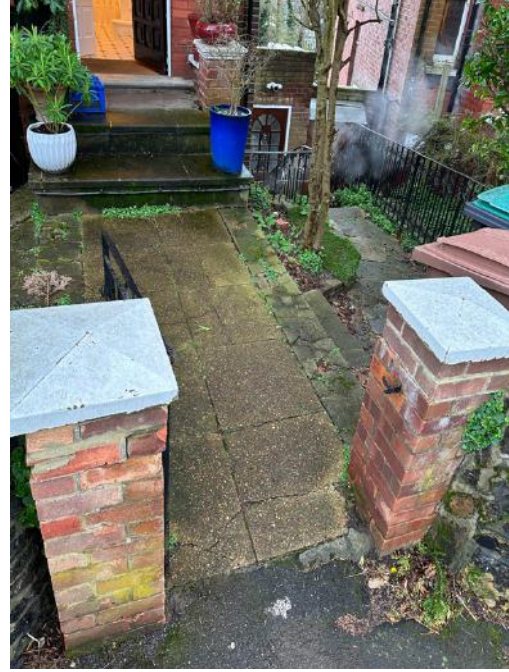
5. Photograph of Existing brick piers and tree to be removed from Front Garden
