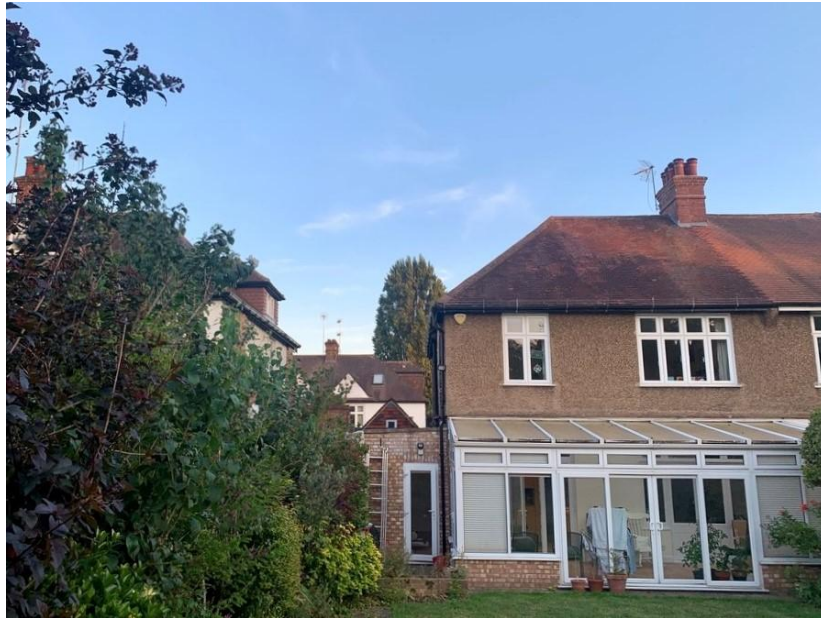
2.2 Rear of 57 Fordington Road as existing, showing disparate elements of conservatory, side extension and garage.
