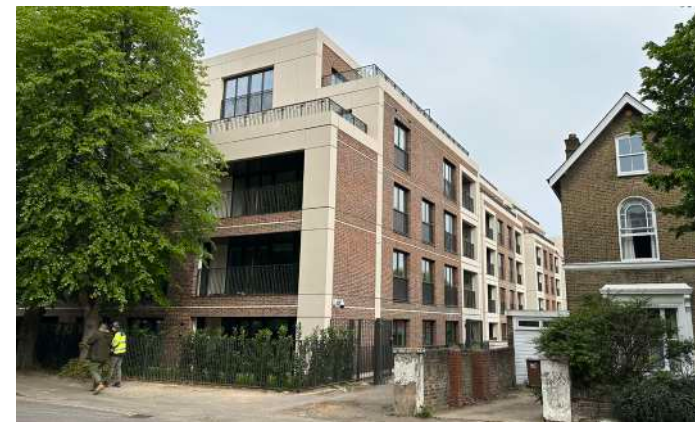
03. Hornsey Town Hall (Housing development under construction 2021-2023)
