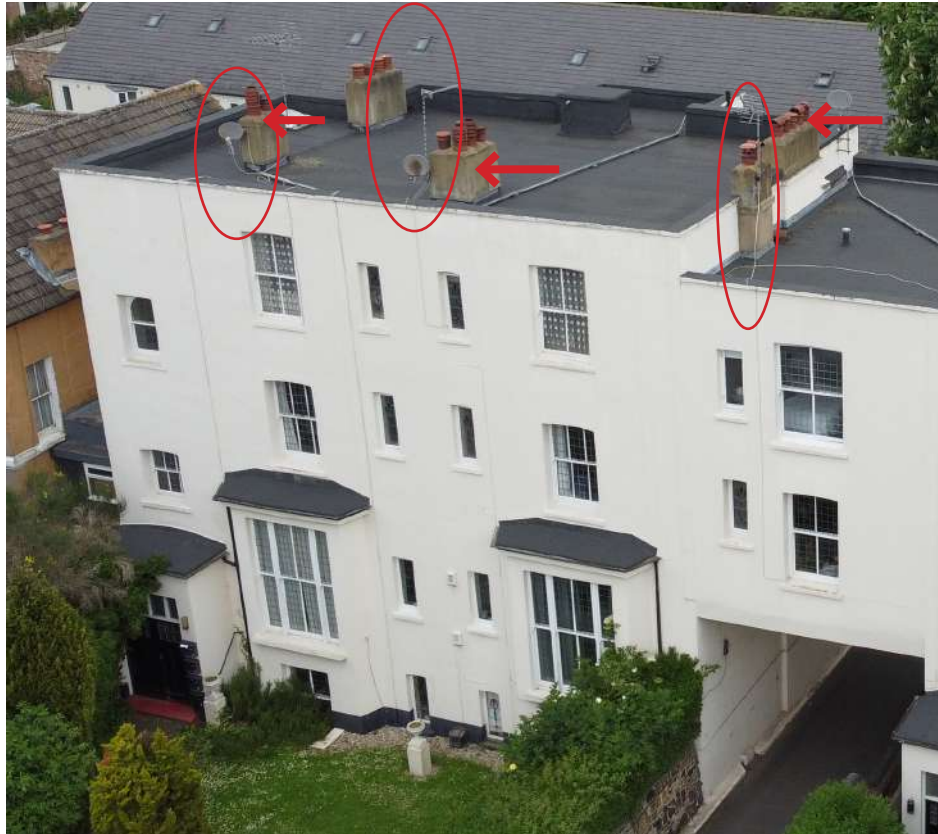
a. Chimneys are finished in a sand cement render which can be seen from street level and aerials and satellite dishes have been fixed close to the front elevation.
