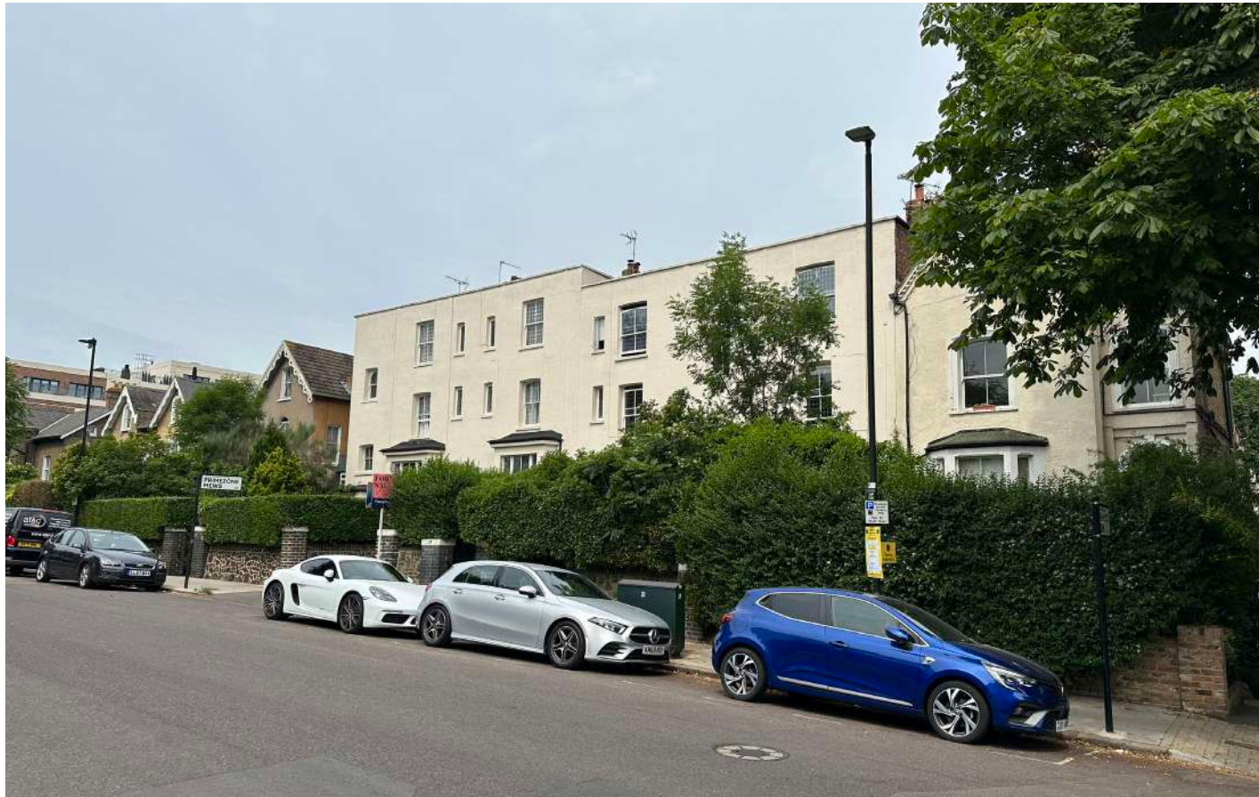
Harcourt House, looking West
