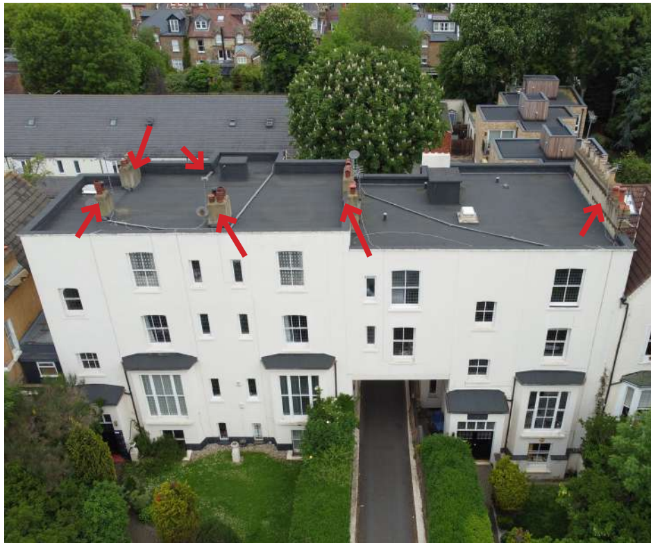
a. Chimneys are finished in a sand cement render which can be seen from street level and aerials and satellite dishes have been fixed close to the front elevation.
