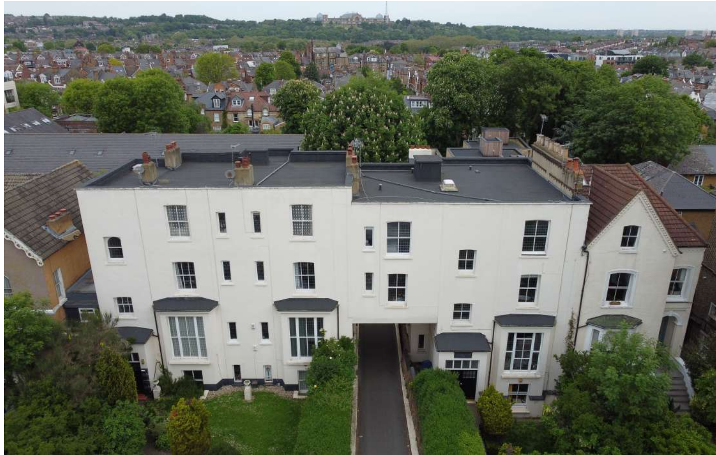
Harcourt House - aerial view of front elevation
