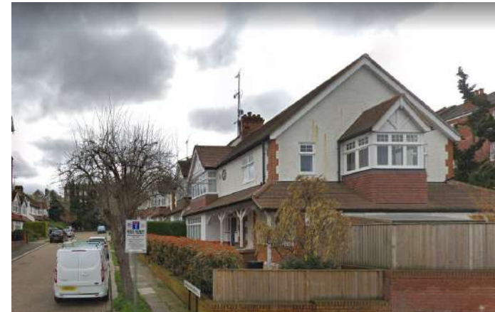
01. View down Sandringham Gardens (2-storey semi detached houses)
