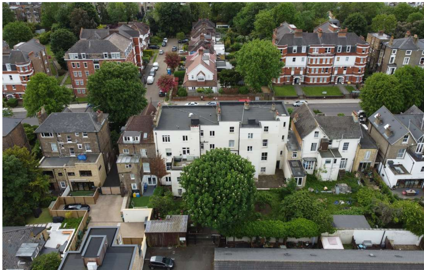
Harcourt House - aerial view of rear elevation, including some neighbouring buildings
