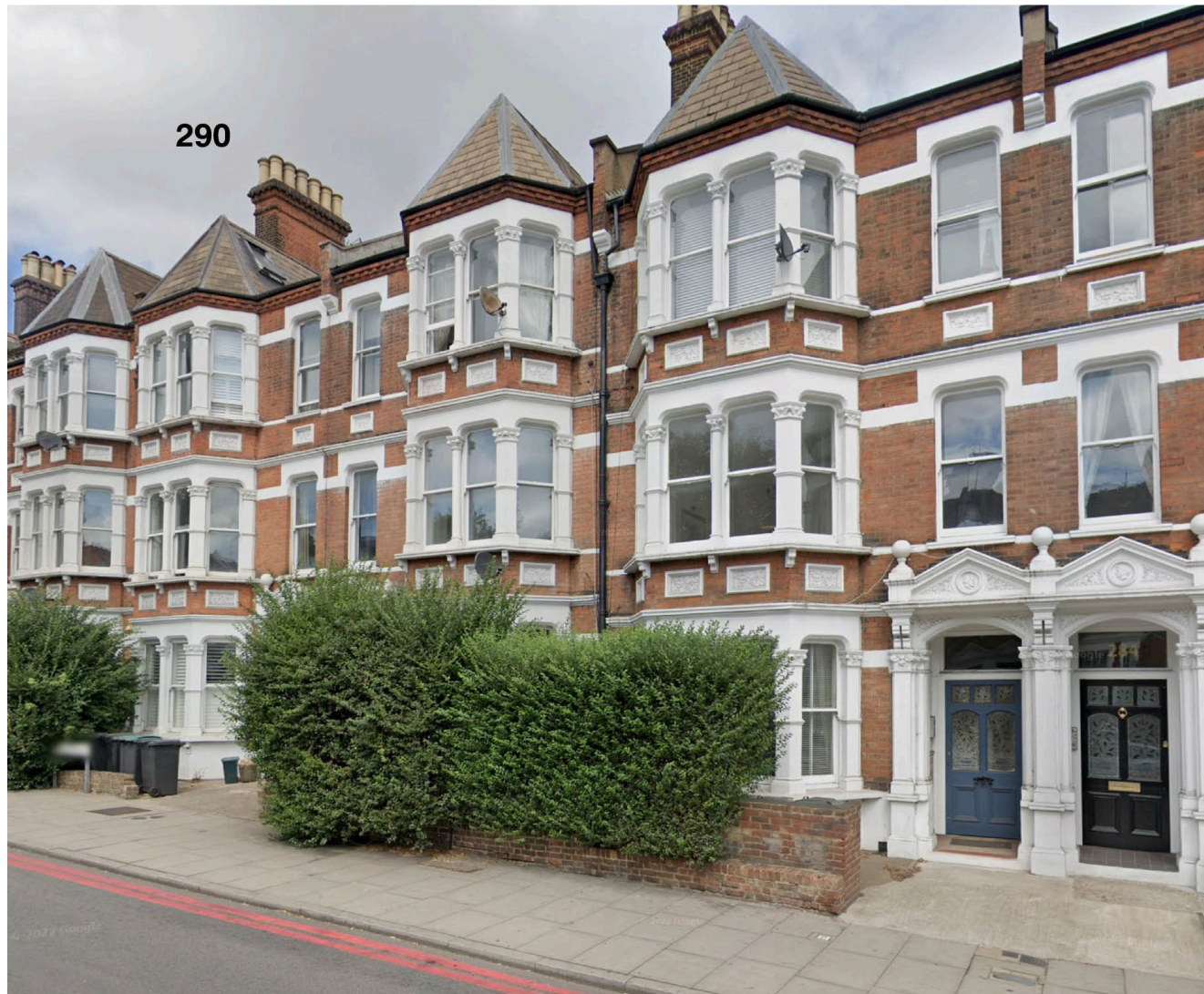
Velux windows in roof 290 Archway Road
