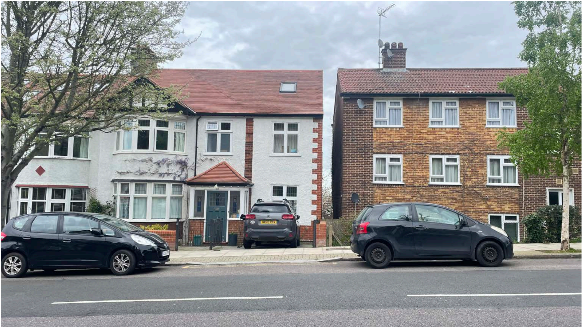
Front Elevation of existing house
