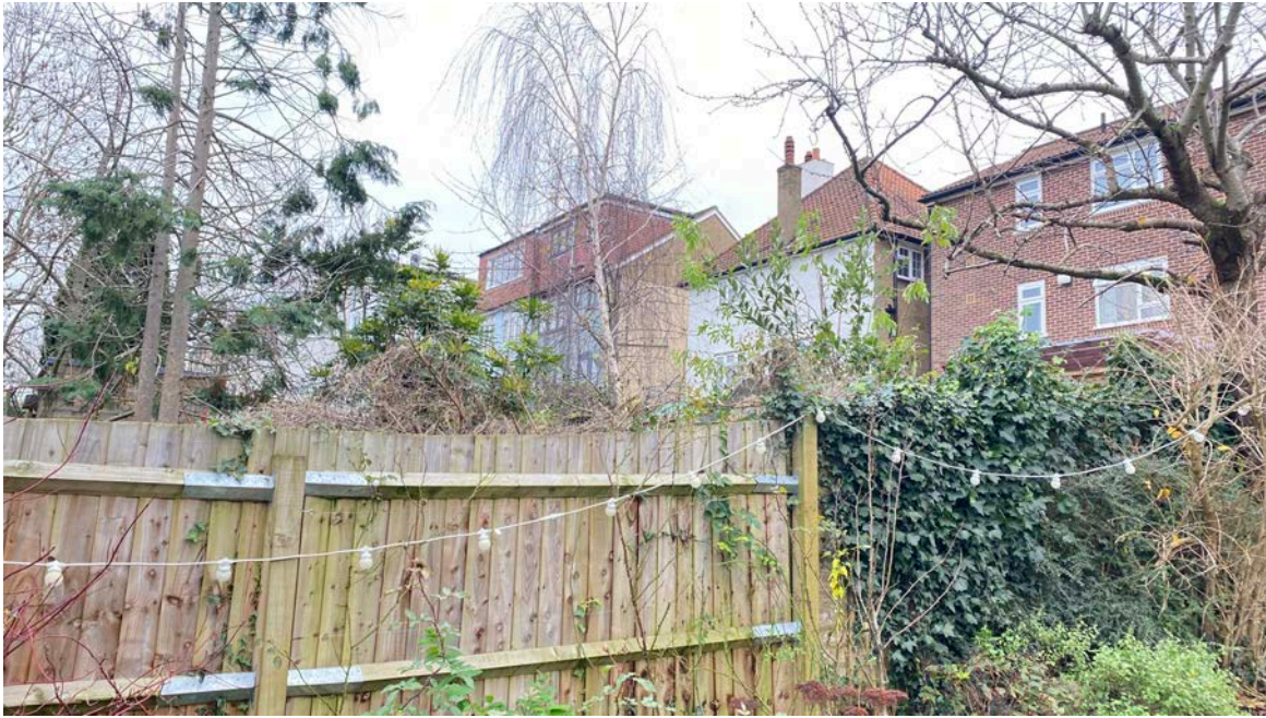
Rear Elevation of Neighbouring property
