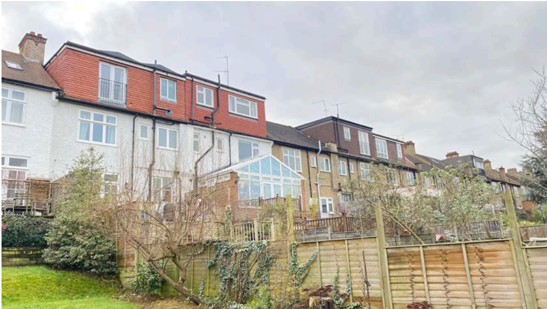
Rear Elevation of Neighbouring property
