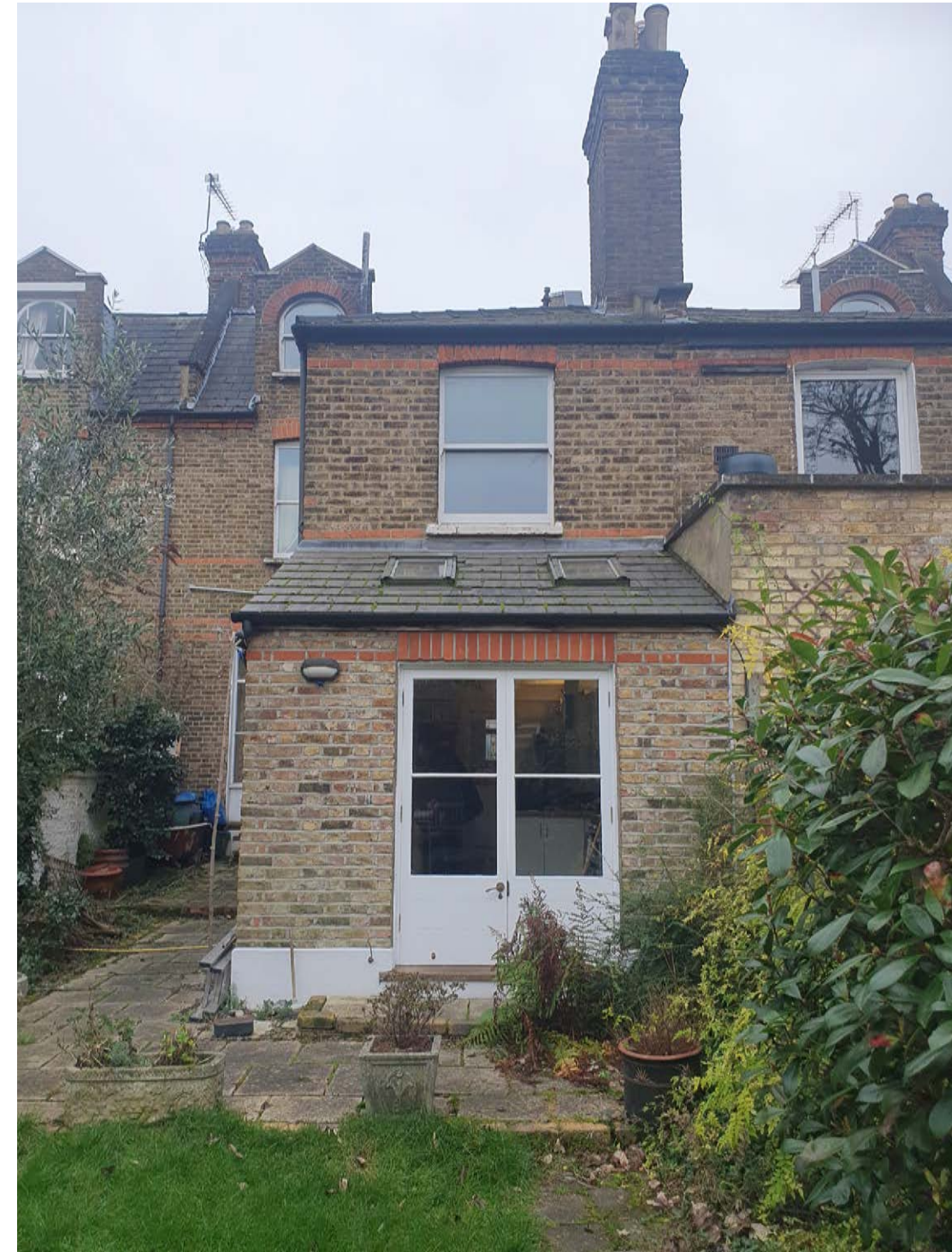
FIGURE 05. Rear Elevation of No.76 Weston Park
