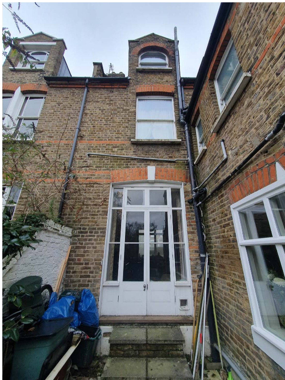
FIGURE 06. Existing Doors from Back Reception Room to be retained
