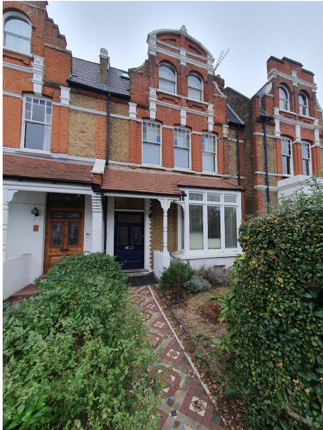
FIGURE 04. Primary Street Facing Elevation of No.76 Weston Park
