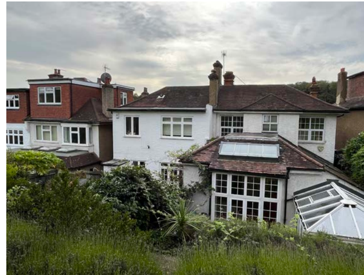
Rear view from the NW
