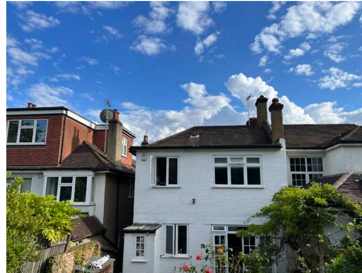
Rear view from the North
