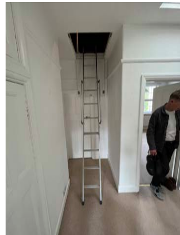
Ladder up to attic space
