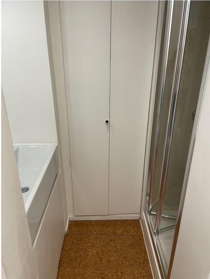
Recess for basin to be blocked up; shower removed
