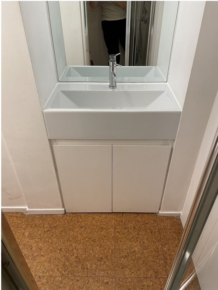
Recess for basin to be blocked up
