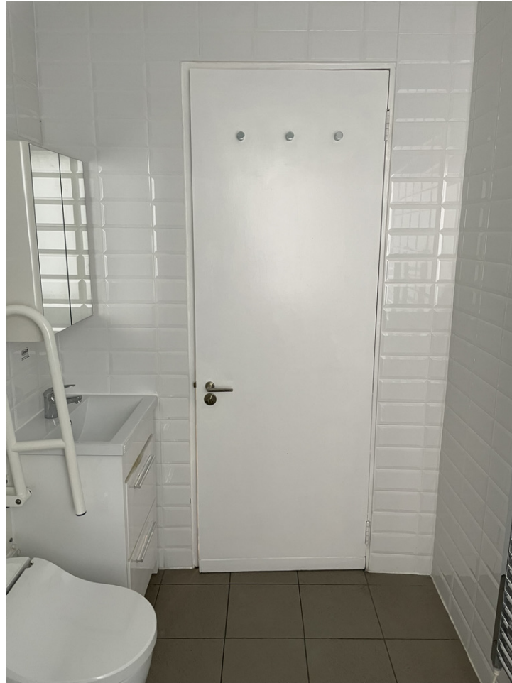
All non-original bathroom fittings to be removed
