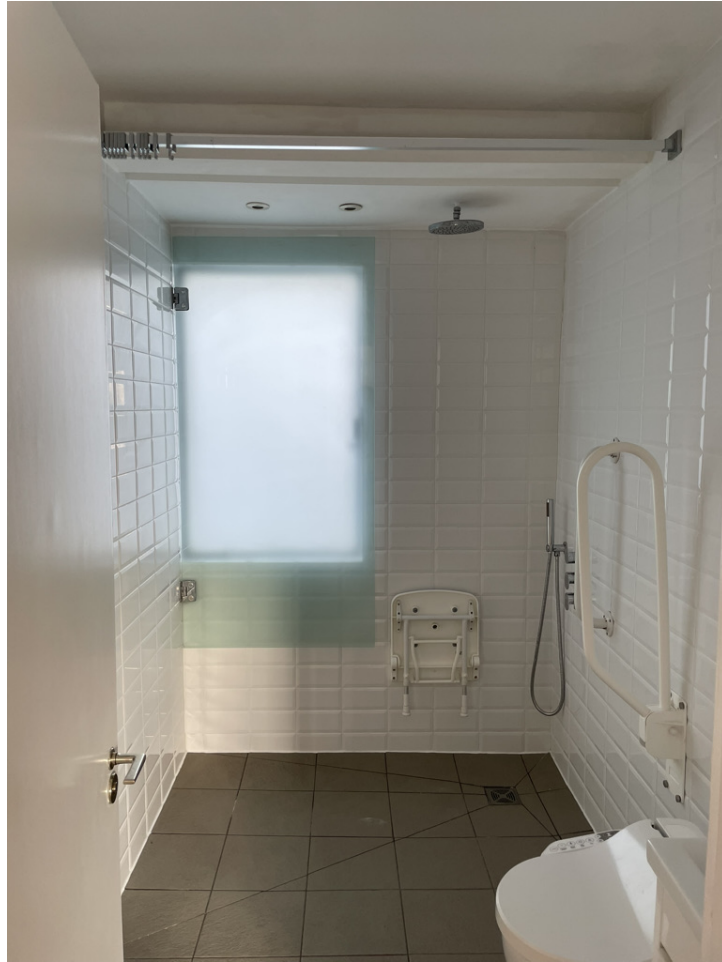
All non-original bathroom fittings and dropped ceiling panel to be removed
