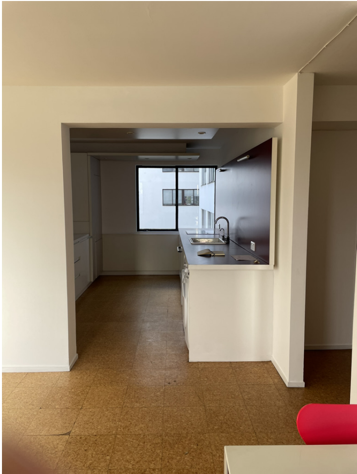
Existing Kitchen - proposed to be reinstated as Dining
