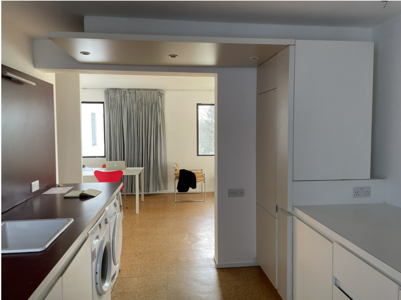
All Kitchen units and dropped ceiling panels to be removed
