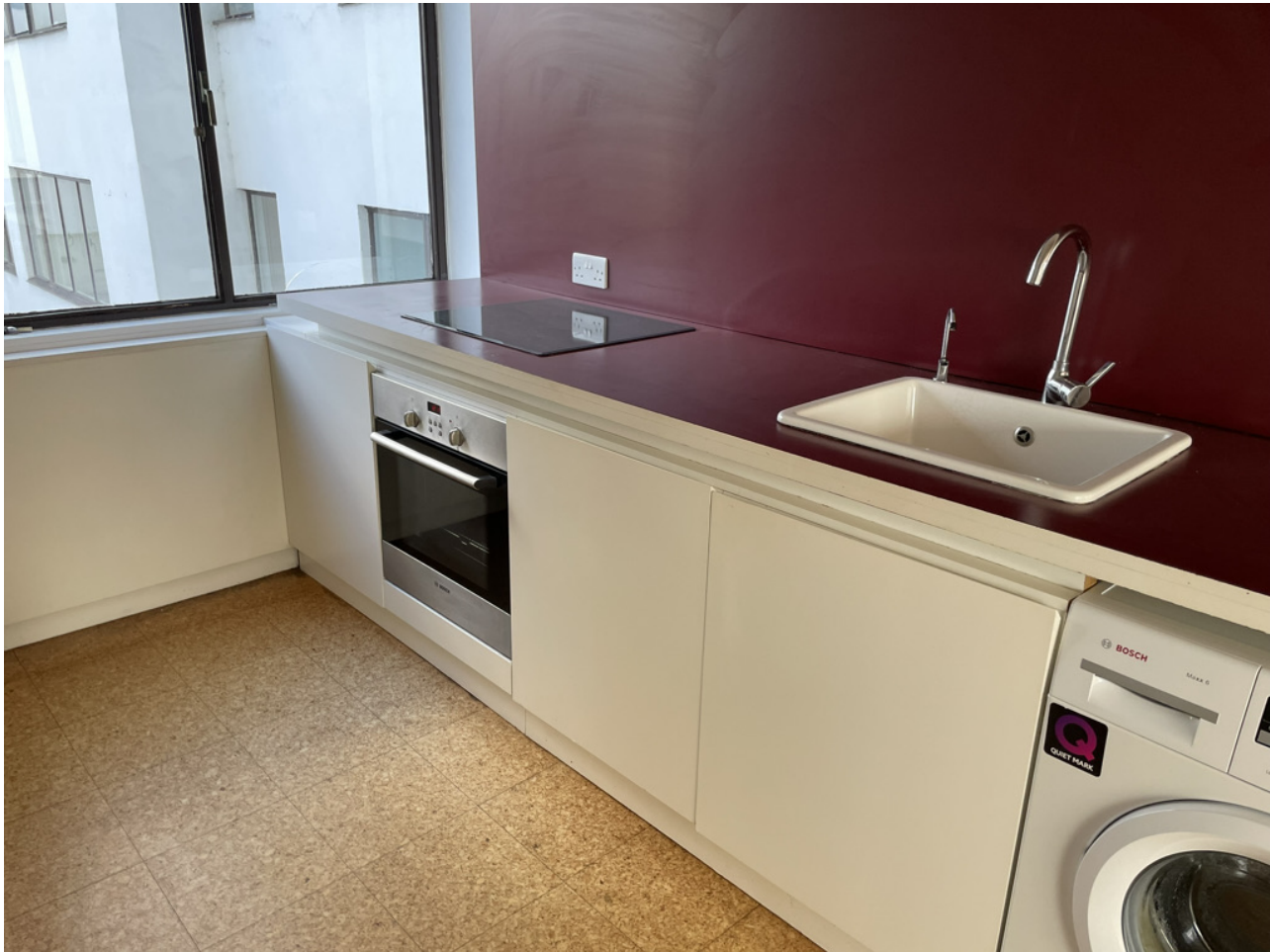
Kitchen units and back panels to be removed
