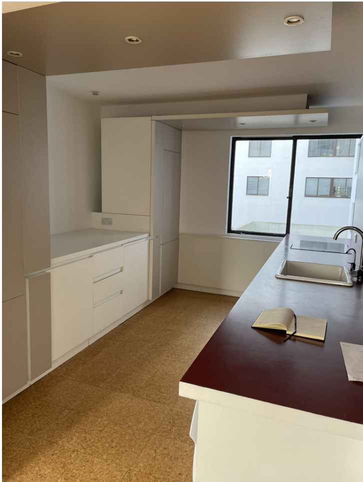
Kitchen units and dropped ceiling panels to be removed
