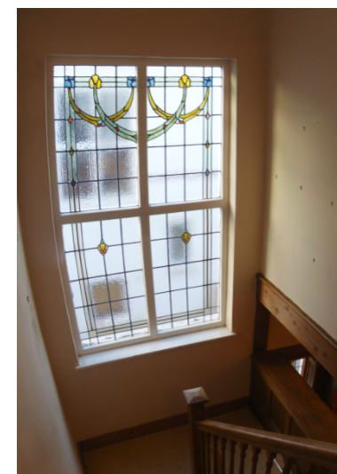
Ground to 1 st floor stairwell.
