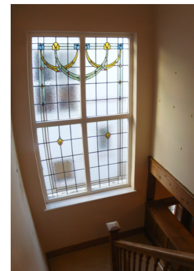
Ground to 1 st floor stairwell.
