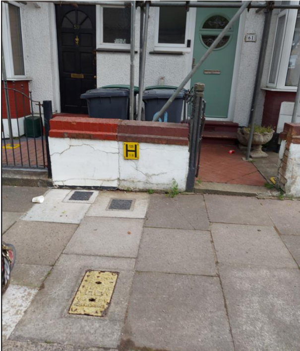
Fire Hydrant Position: 59/61 Keston Road (opposite site).
