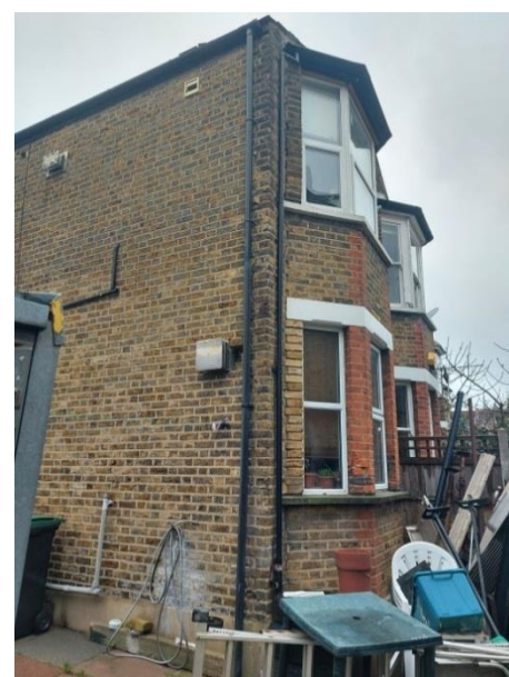
Rear elevation (Bay end).
