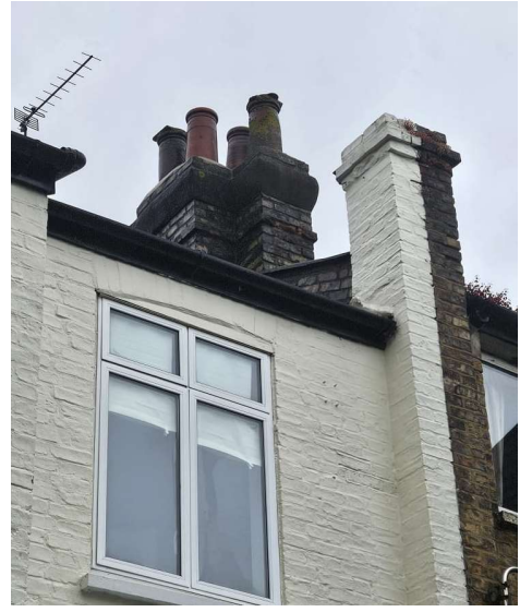
Fig 3. Photo of existing chimney breast
