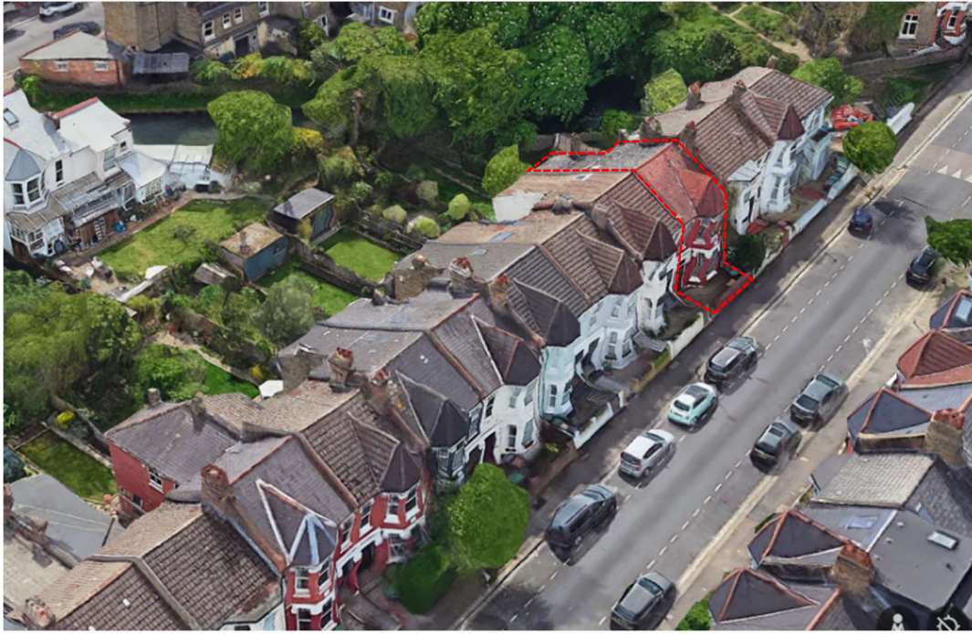
Fig 2. Aerial view looking south-west from Seymour Road
