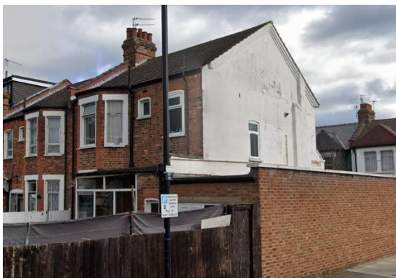
105 Boundary Road – before
