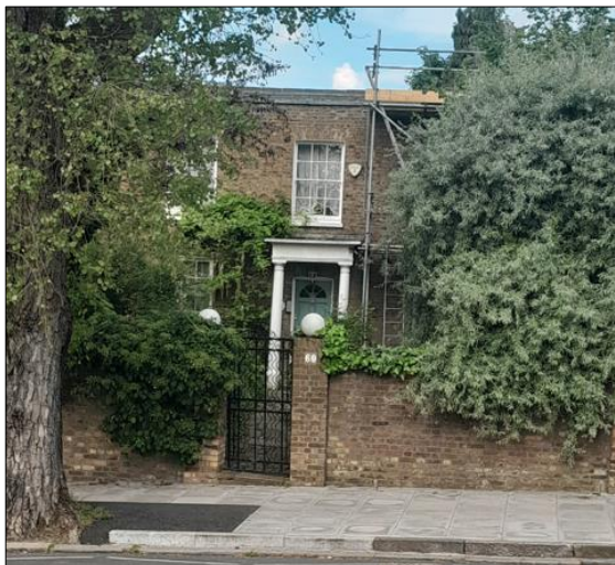
Figure 11. No.60 North Hill. Street elevation of asset, facing west onto North Hill.
