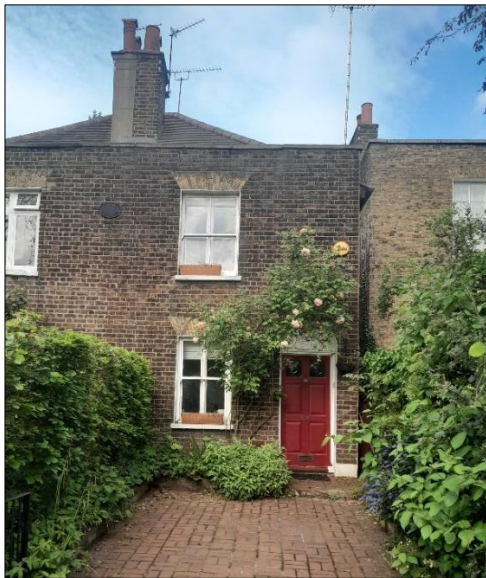
Figure 1. Subject property. Street facing elevation. Image taken: 18th May.
