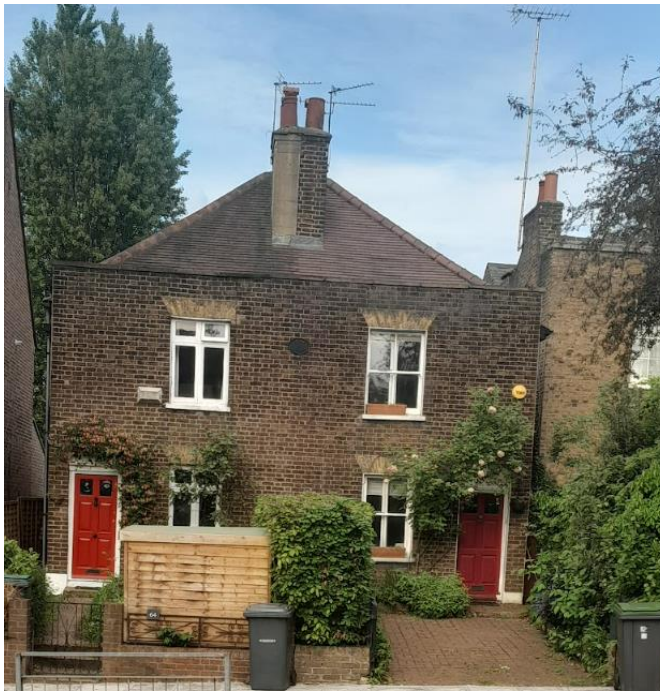
Figure 3. Principal (west) elevation of 62-64 North Hill
