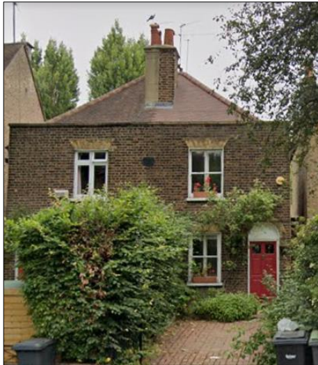
Figure 8. Street (west) elevation of asset: May 2023.
