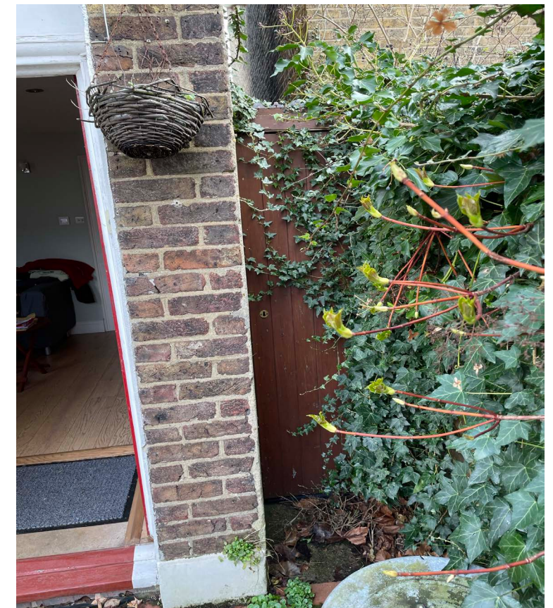
PHOTO 03 - FRONT VIEW OF SIDE CORRIDOR
