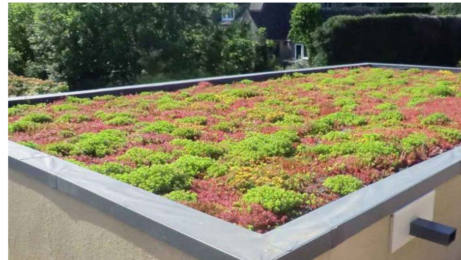
SEDUM GREEN ROOF - LOW MAINTENANCE
