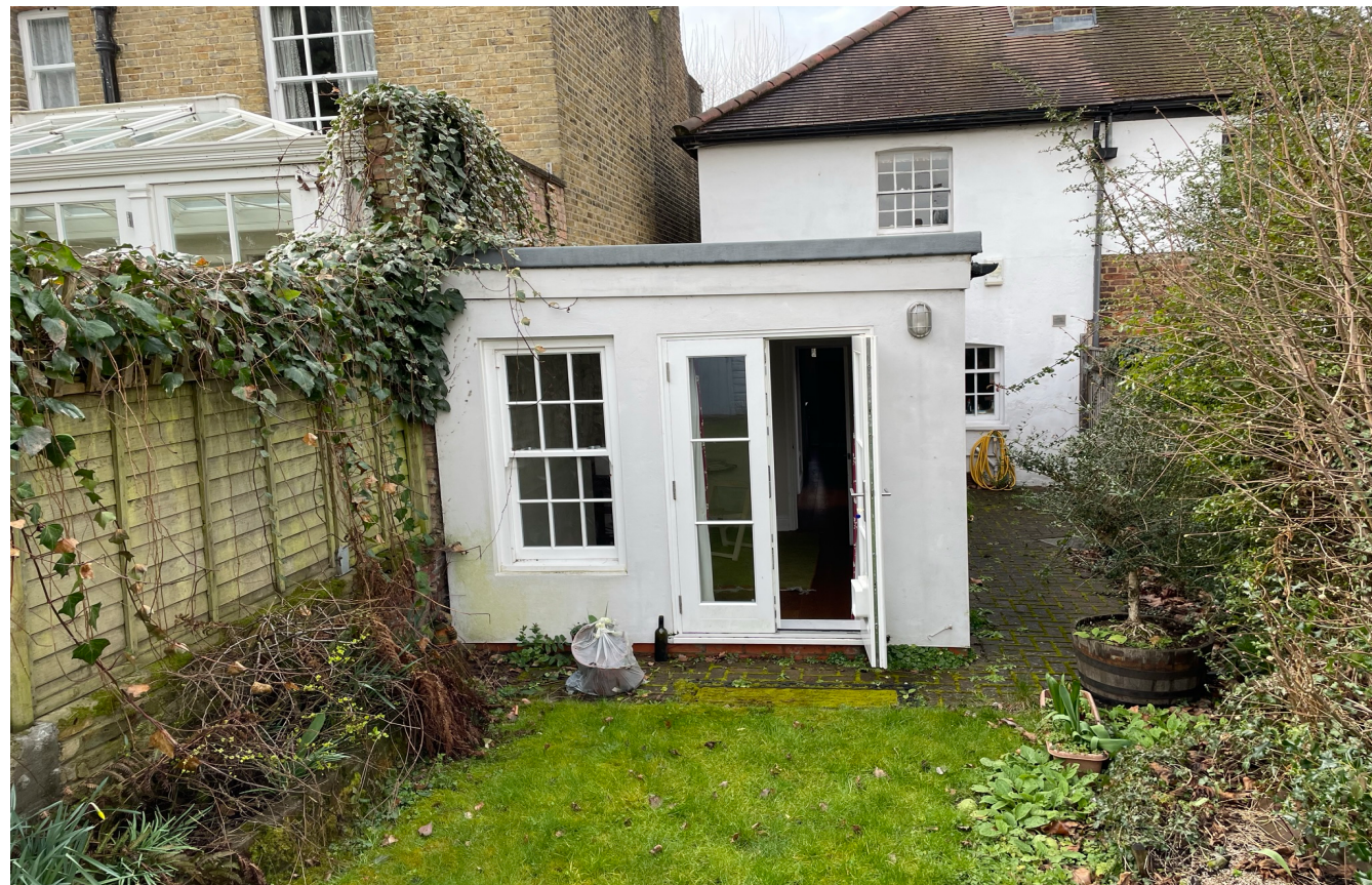
PHOTO 01 - REAR VIEW OF THE COTTAGE EXTENSION
