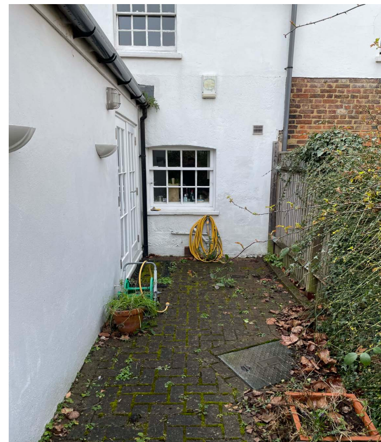
PHOTO 05 - REAR VIEW OF THE COTTAGE
