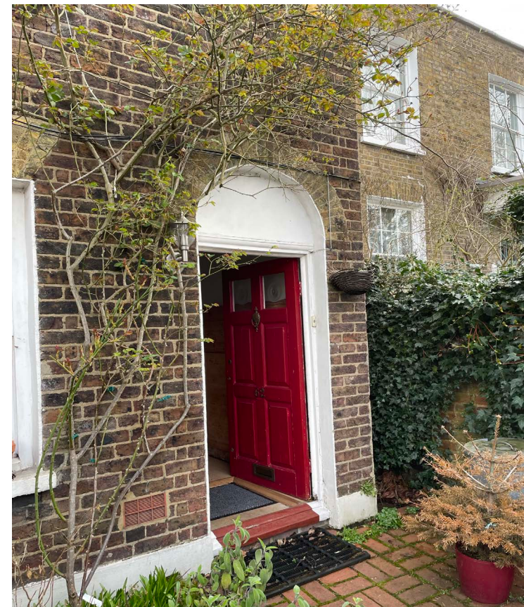
PHOTO 02 - FRONT VIEW OF COTTAGE
